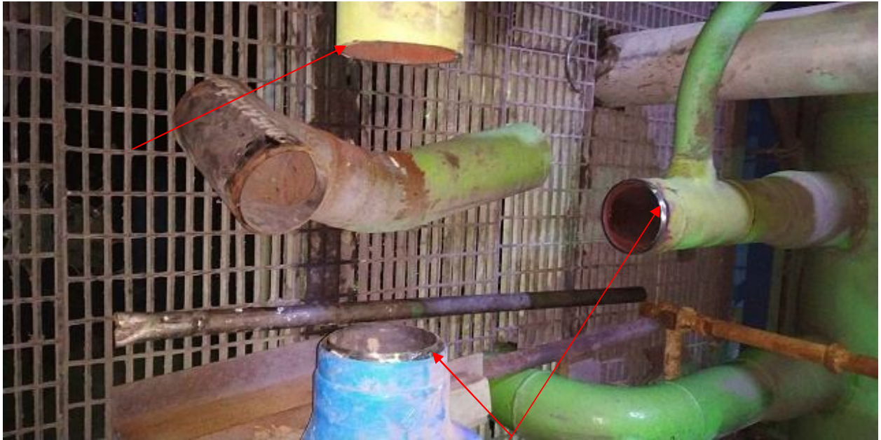
Figure 1: Header cutting done and edge preparation is under progress
