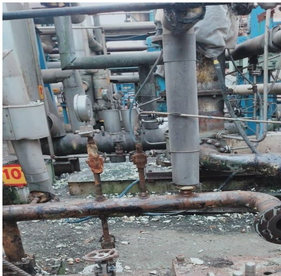
Ammonia Tr pump.drain line pressure gauge nipple welding
