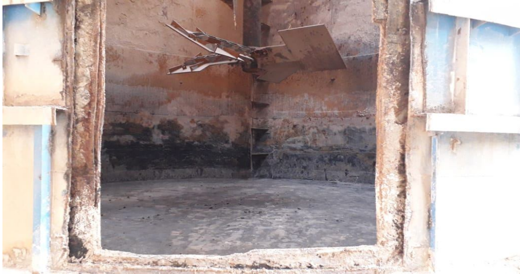
SST after cleaning
