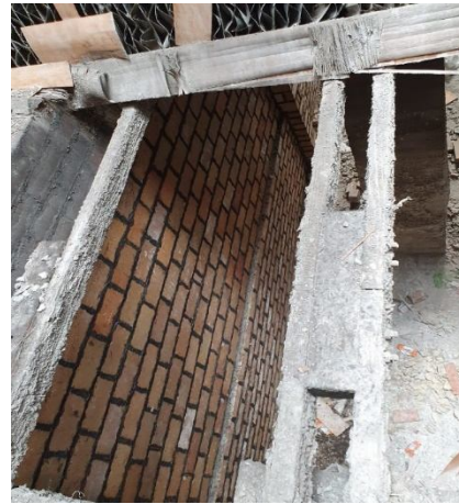
New Cooling Tower cold well cell after repairing
