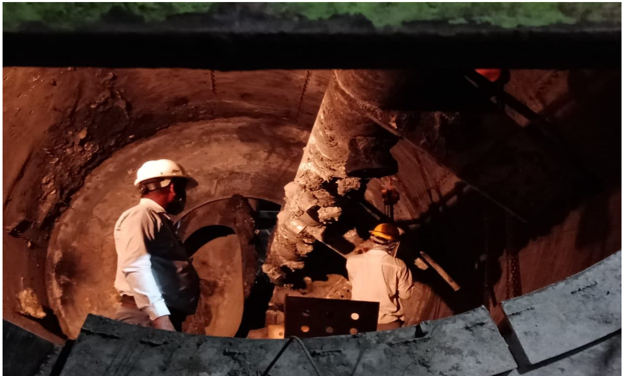
Ammonia sparger replacement
