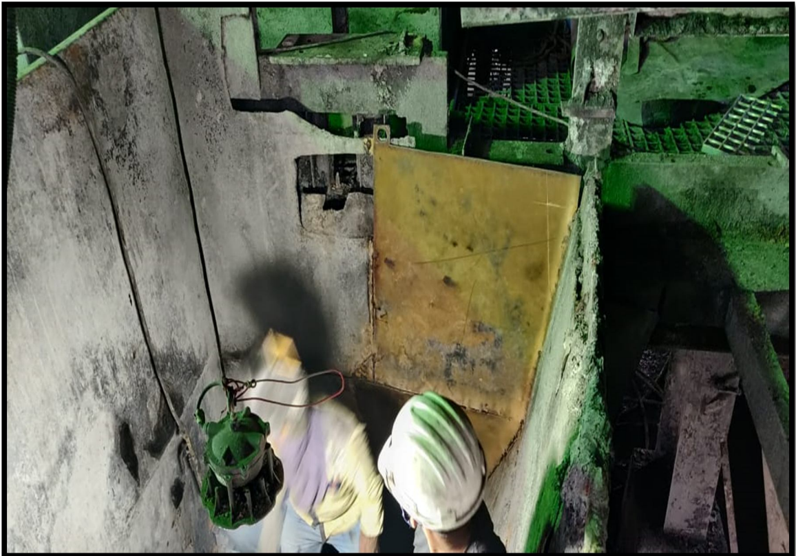
Fines Conveyor discharge hopper repair
