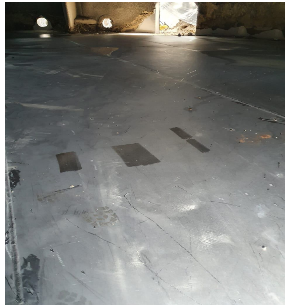
Pump Tank after cleaning
