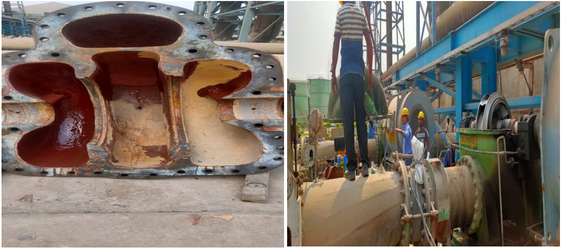
FIG: Pump C casing and Rotor assembly.
