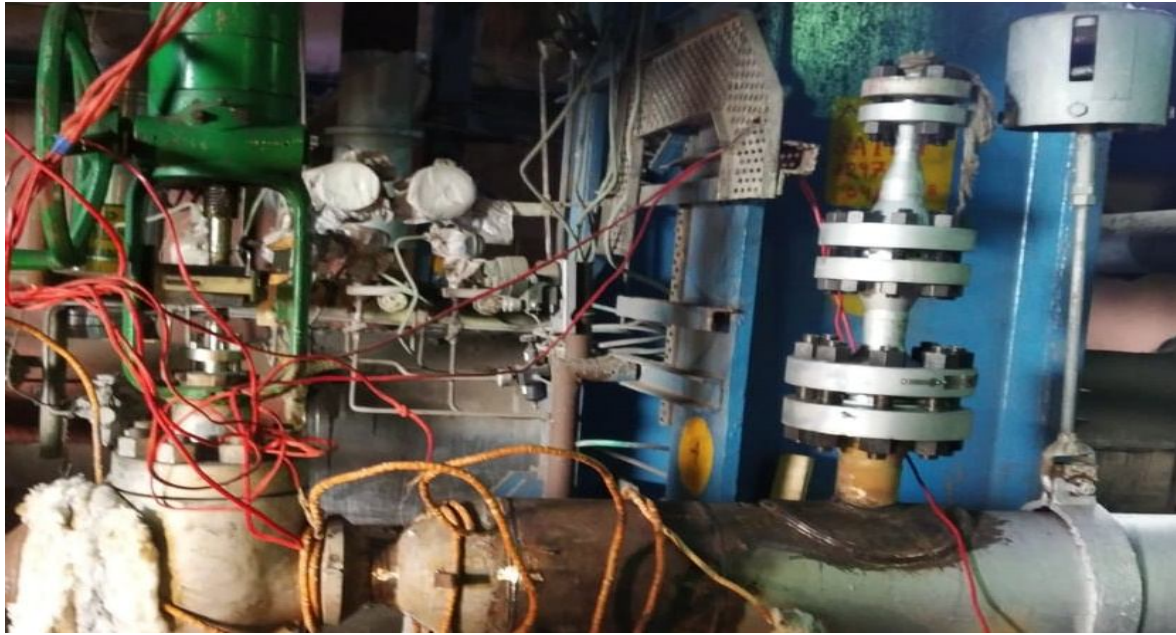
Figure 15: Final welding completed
