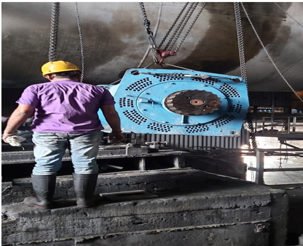
Dryer motor shifting
