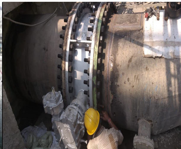
Suction Valve After Replacement
