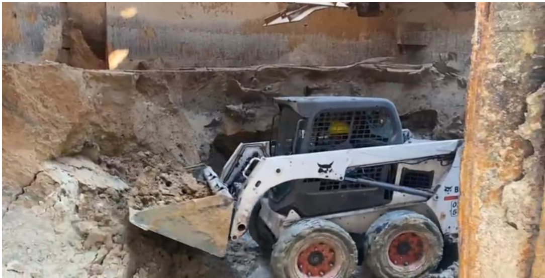
SST Cleaning with skid loader
