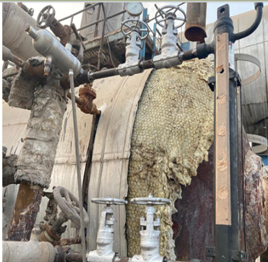
HYDRASTEP INSTALLATION IN SAP-2 BOILER
