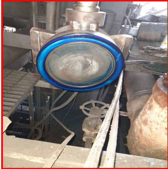
Boiler-2 MSSV overhauling
