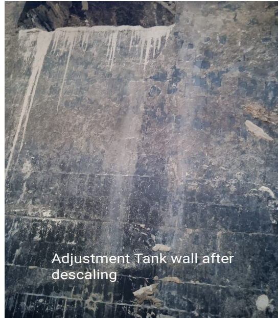
Adjustment tank wall after
