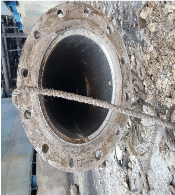
Misc Pipe Line after Cleaning
