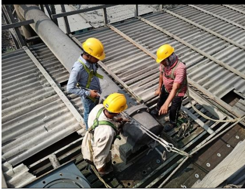
Removal of old FCV
