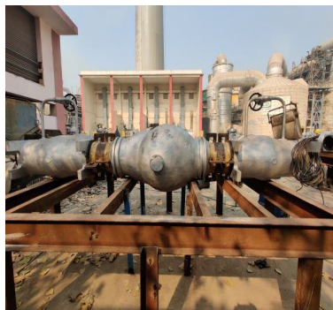
Pre-fabrication of valve assembly
