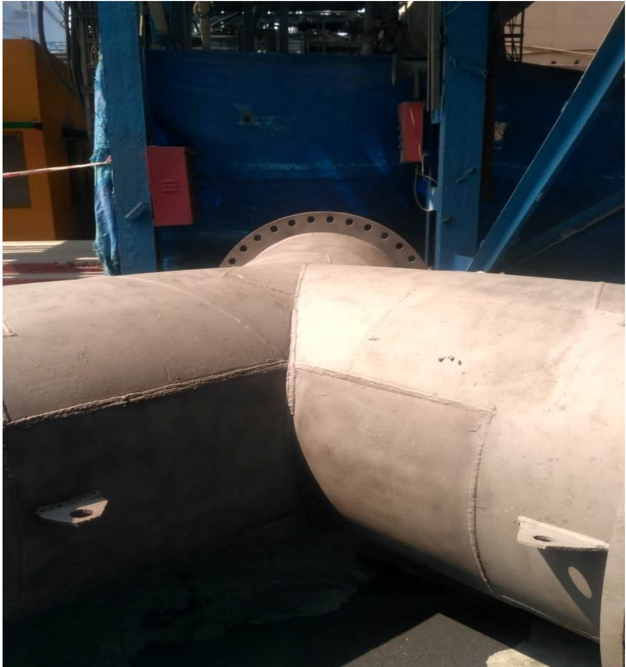
NEW / FABRICATED "Y - PIECE" INSTALLED IN P-113 PUMP DISCHARGE
