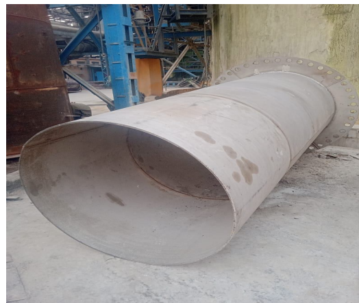
Seal Leg after cleaning
