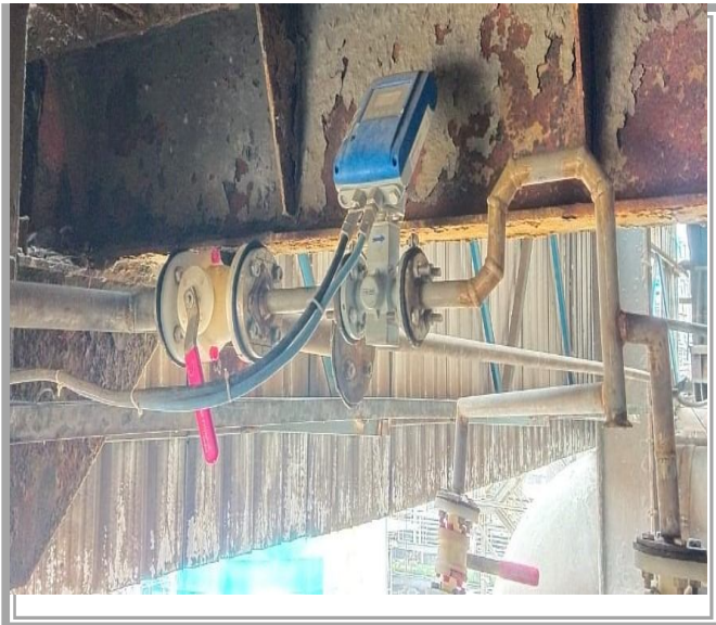
M/s Krohne Marshall make Electromagnetic Flowmeters in Flocculent lines
