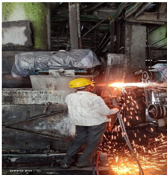
Old casing removal
