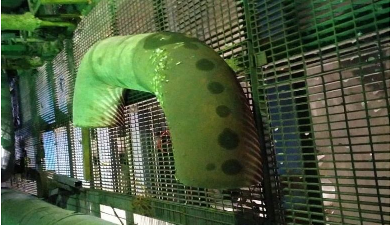
Figure 2: 400 NB LP header portion to be replaced is removed
