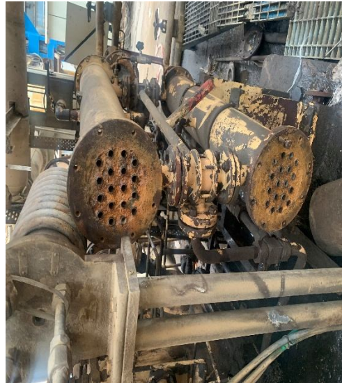
Fig 1.4.1(e) lube oil cooler of bcw turbine before and after cleaning
