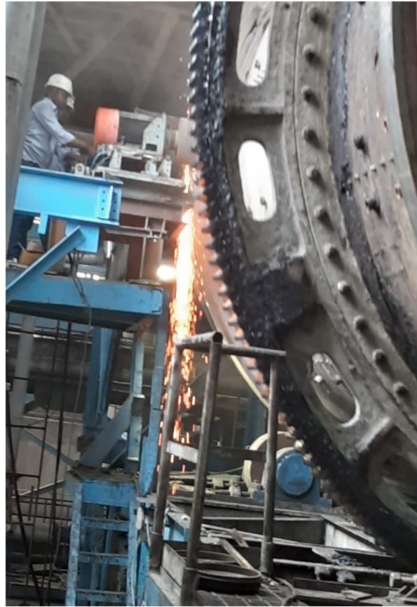
Feed end tyre grinding
