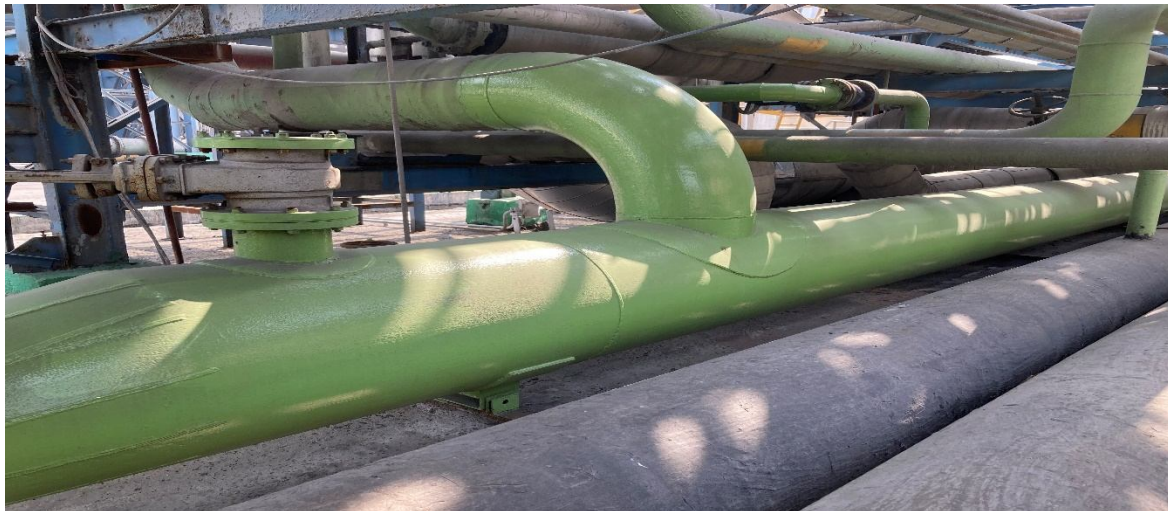
Fig-Filter water line after Replacement
