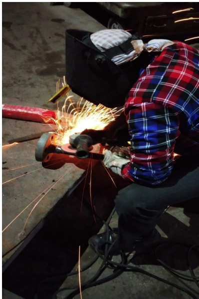
Figure 16: Preparing for TCV positioning
