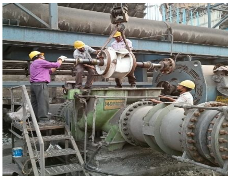
TG CT PUMP S IMPELLER FITTING
