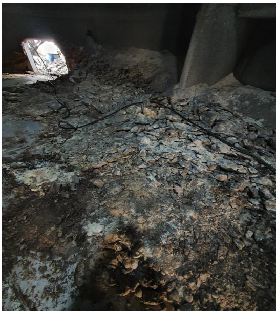
Pump Tank before cleaning
