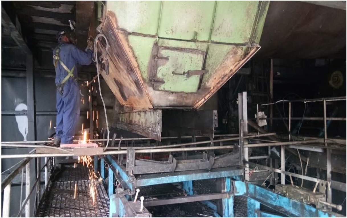
Dryer discharge hopper welding & new plate erection
