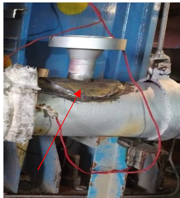
Figure 6: Branch joint pad fitted
