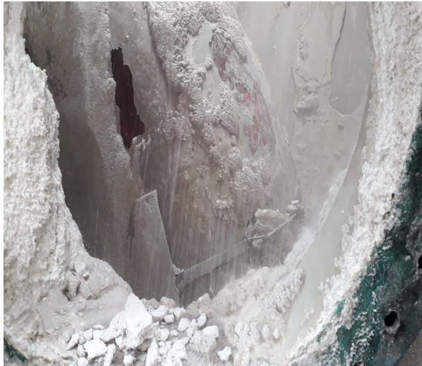
Pre scrubber bottom cone before cleaning
