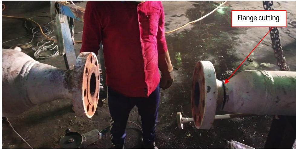
Figure 1: Old PCV removed and flange cutting started
