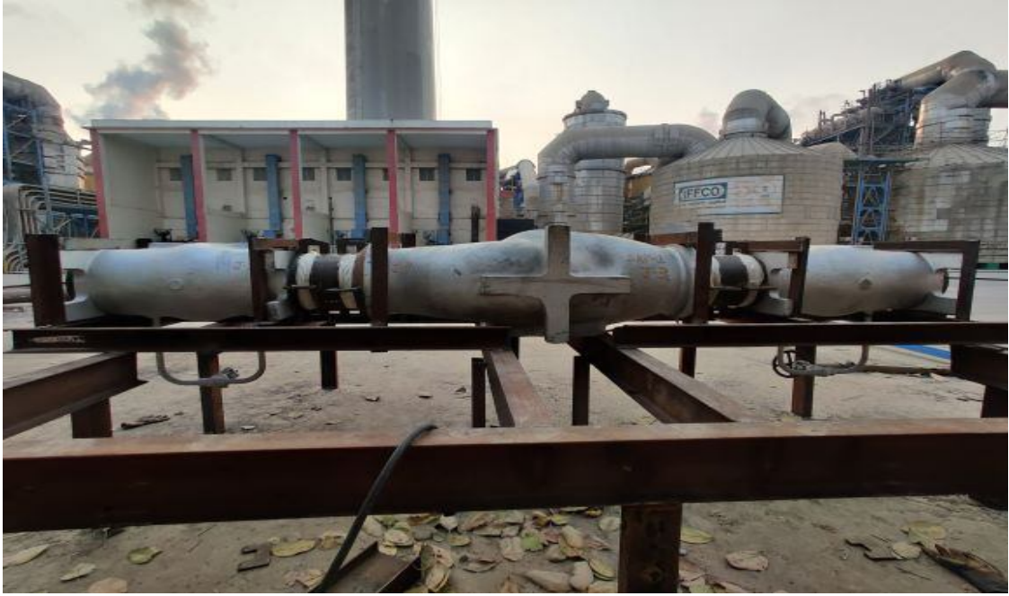
Pre-fabrication of valve assembl
