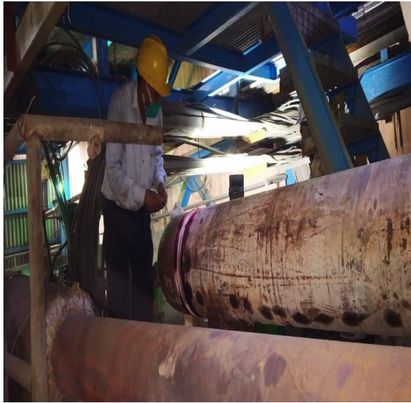
Figure 11: DP test for Joint-2 root welding
