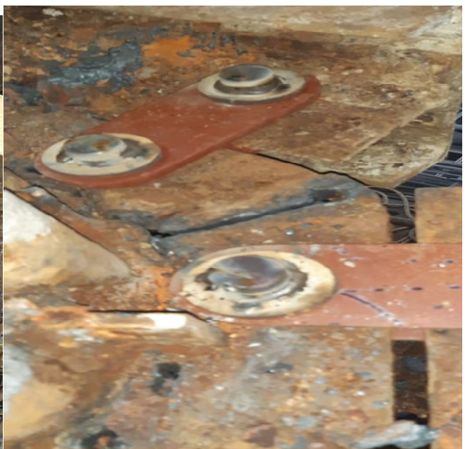
Various pictures of Buck stay corner plate modified at various elevations
