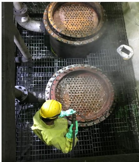
Cooler tubes cleaning
