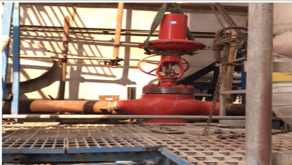
New Drum level Control Valve Tag 10LCV2301
