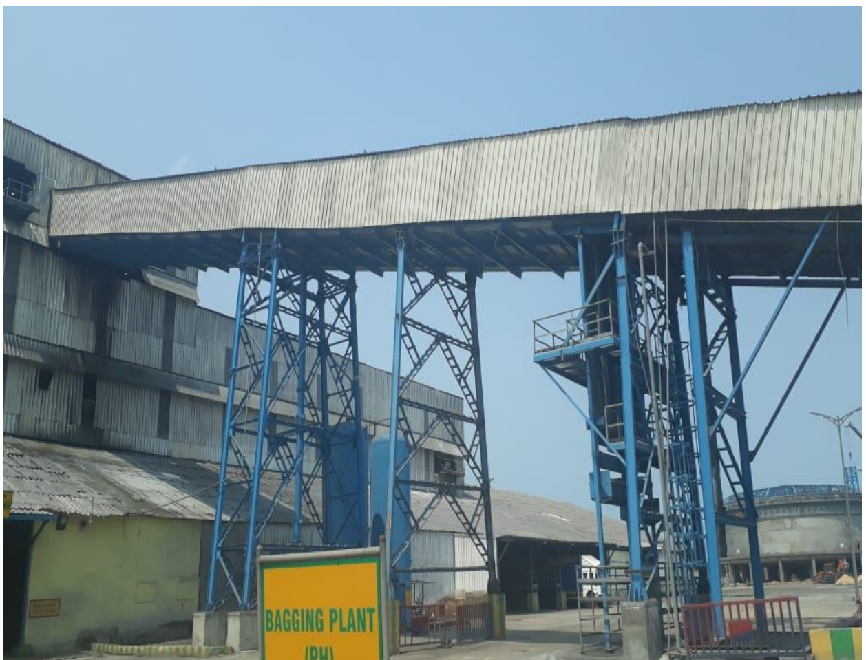
ALL NEW GALLERIES – 1 & 2 ALONG WITH TRESTLE NO-1 & 3 AFTER ERECTION:
