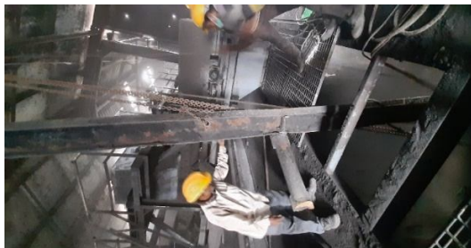
DAMAGED BEAM REMOVAL WORK
