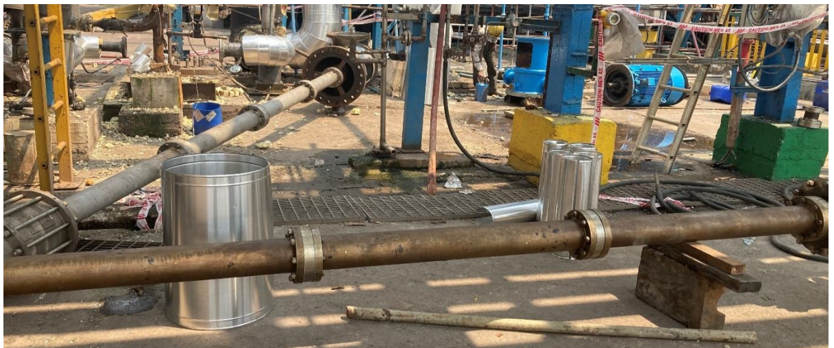
Ammonia Transfer pump-A Ready or Erection.
