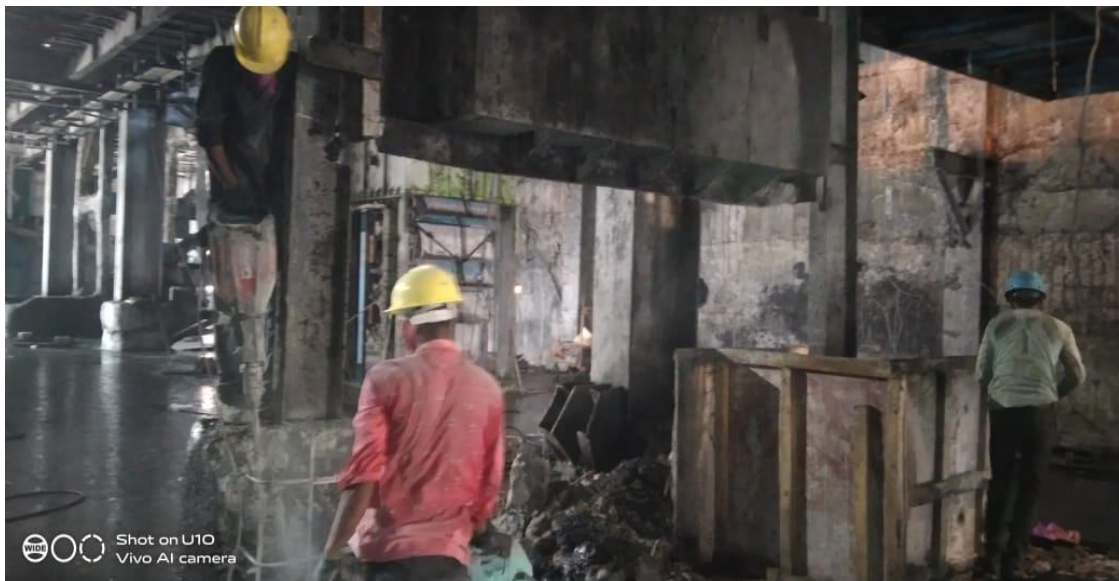
Take up column grouting New stand
