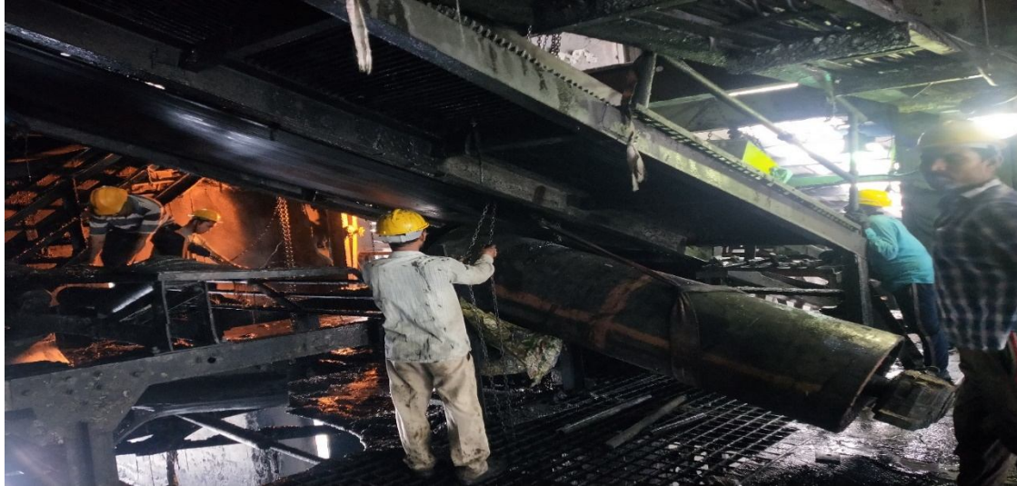
Tail pulley shifting
