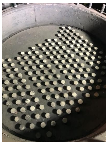
After sand blasting
