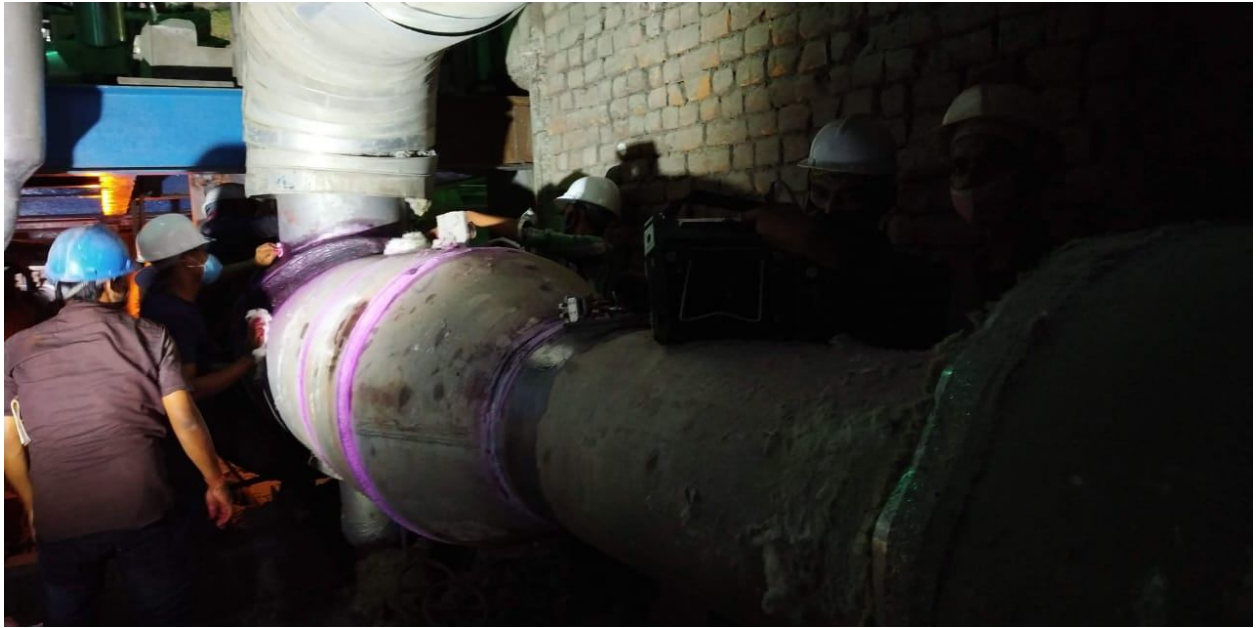
Figure 4: Testing of joints under progress
