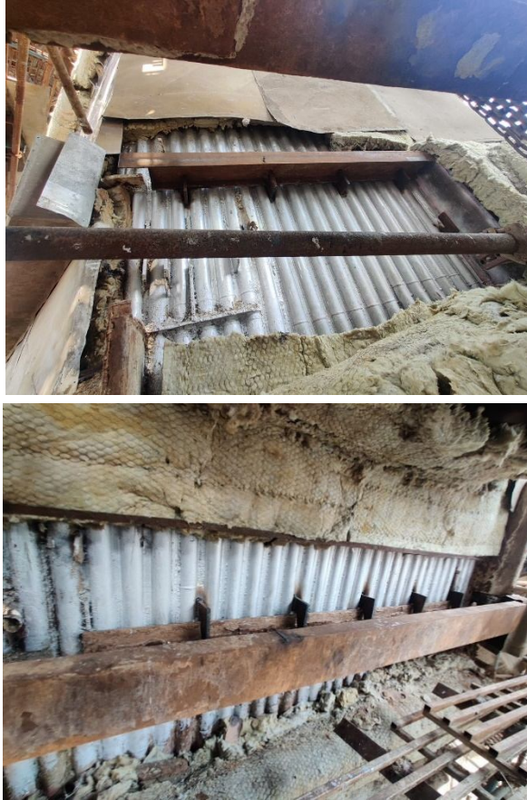
Replacement of Expansion Bellow at Boiler Bypass duct – 1800 NB
