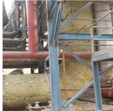
LPS2 Header Insulation
