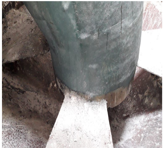
Pre scrubber bottom cone after cleaning
