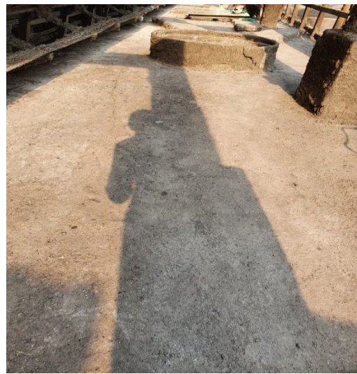
Cooling Tower deck after cleaning
