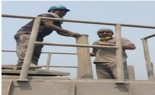
OLD BAGS WITH SS CAGE REMOVING WITH CAGE ARE LIFTING
