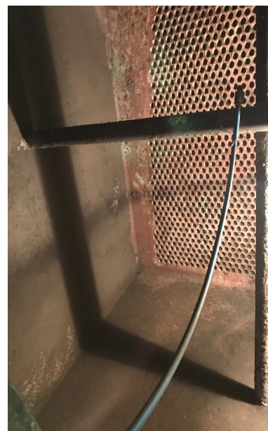
After sand blasting
