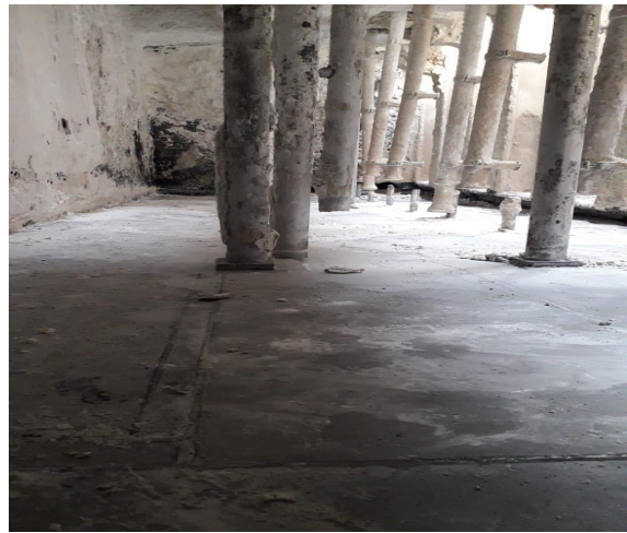
Fumes Scrubber chamber after cleaning
