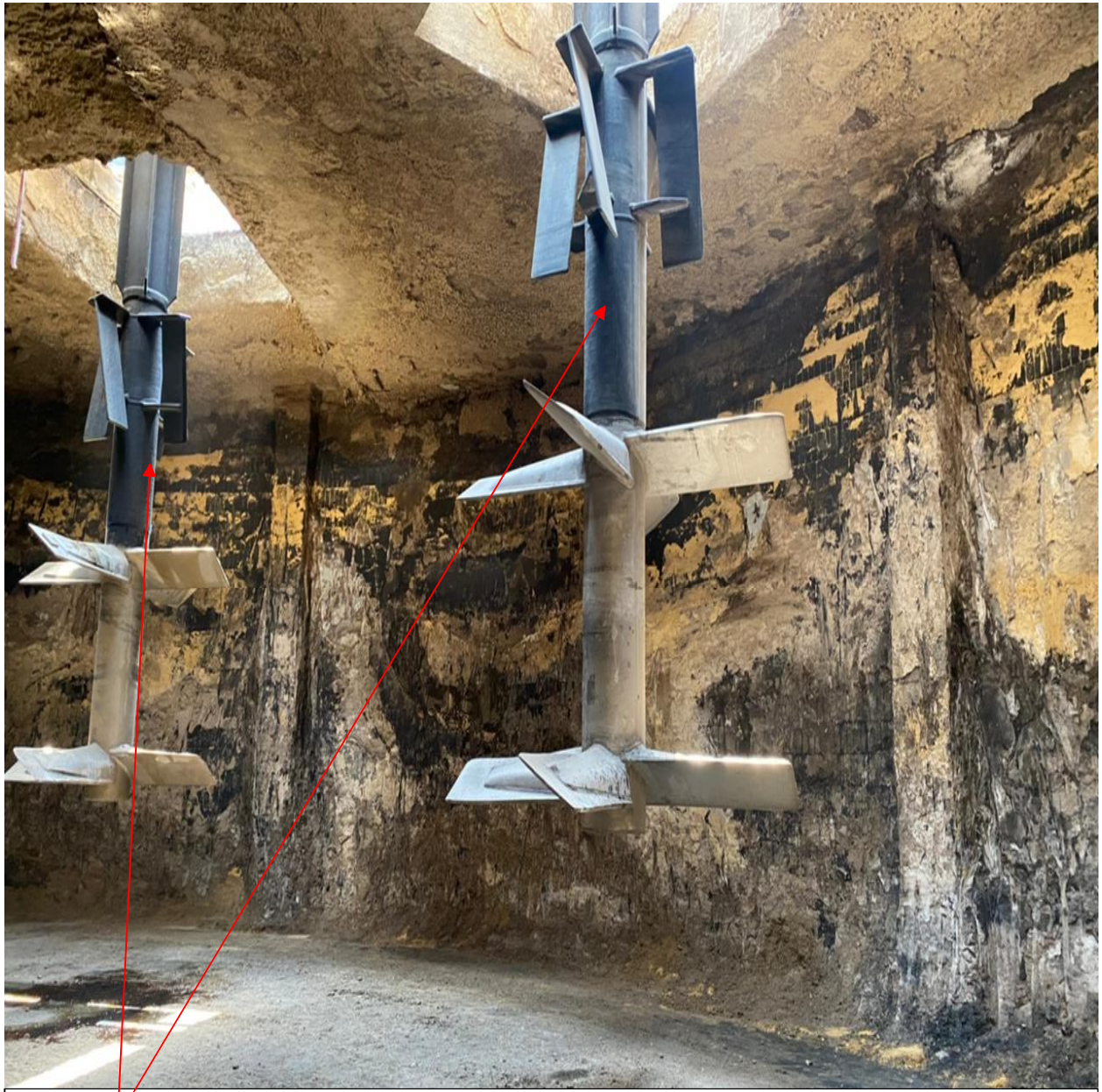
REPAIRED SPARE AGITATORS INSTALLED IN 05-111 & 05-112 LOCATION IN ANNULAR COMPARTMENT.
