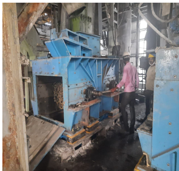
New casing erection
