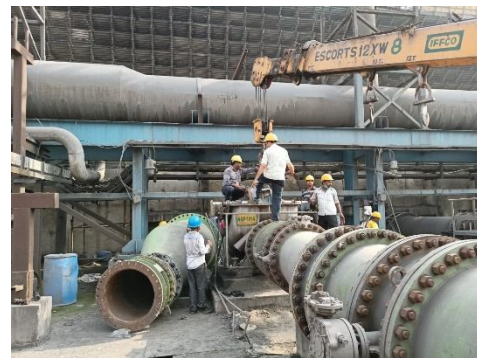
TG CT PUMP S IMPELLER FITTING
