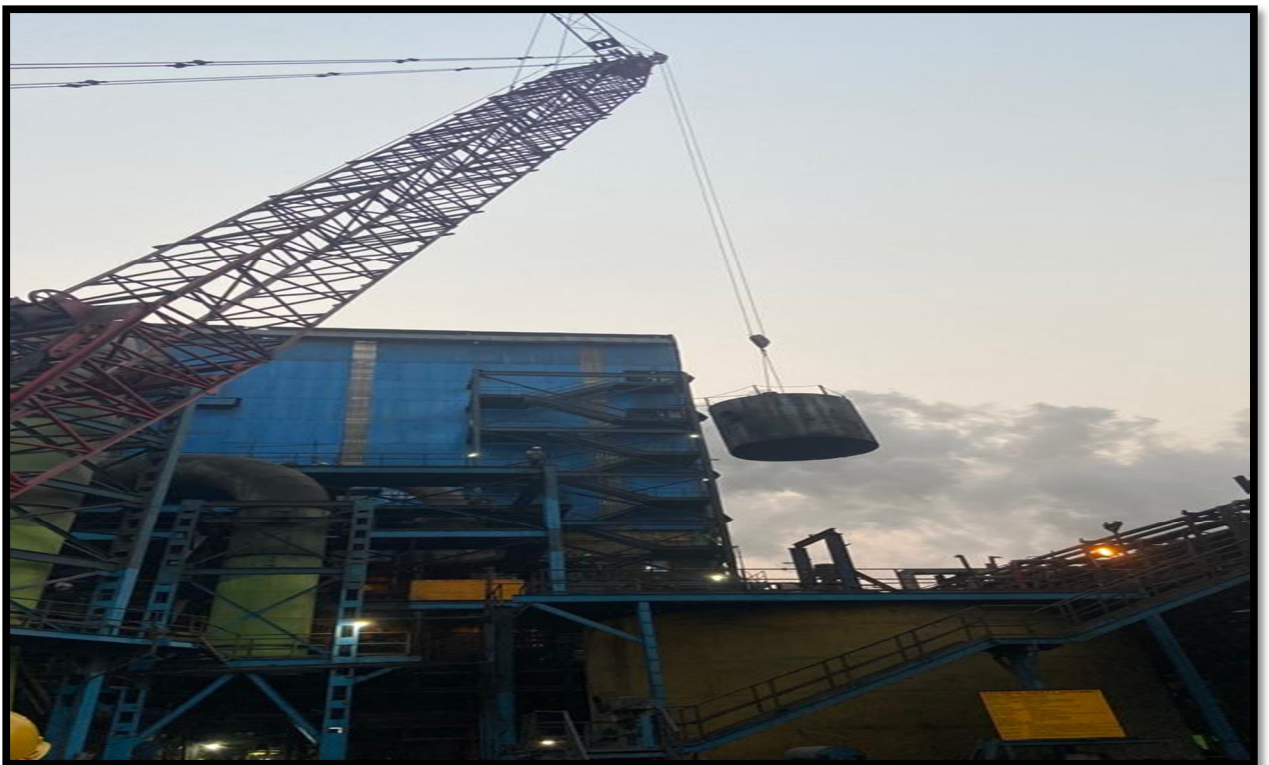
Erection of Pre Scrubber shell
