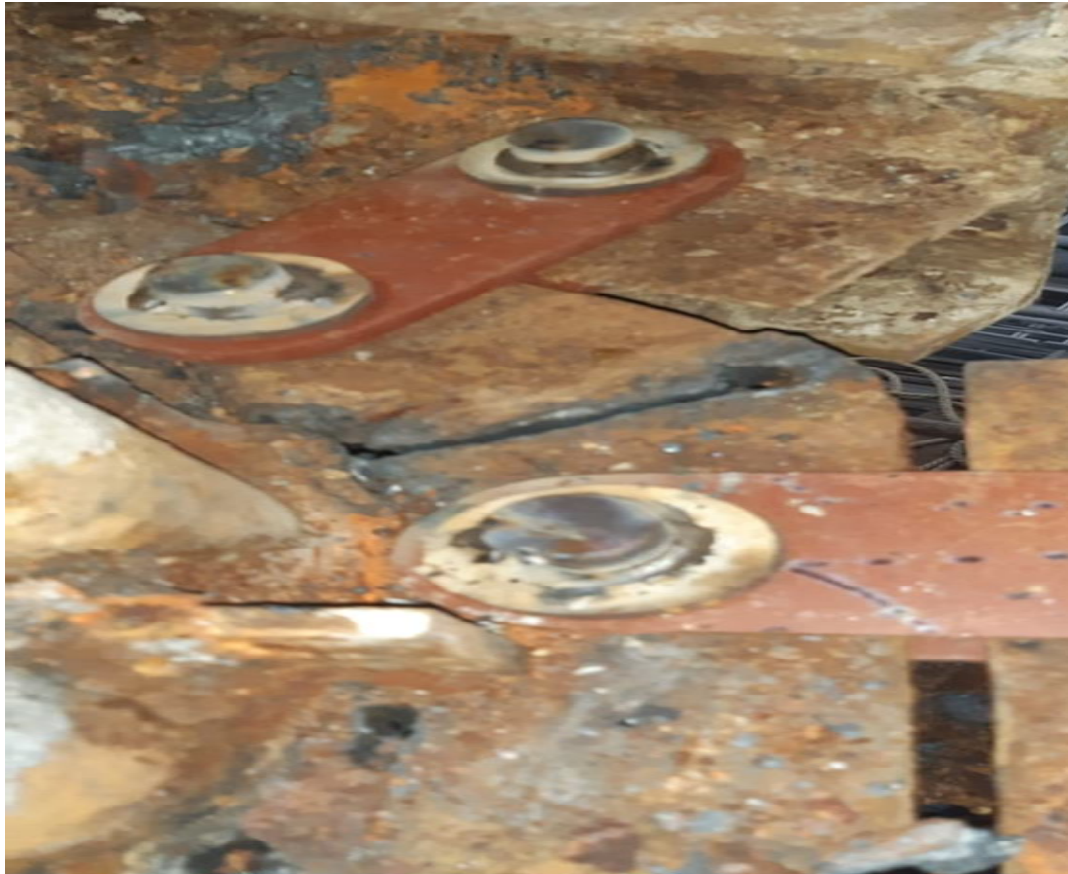
Various pictures of Buck stay corner plate modified at various elevations
