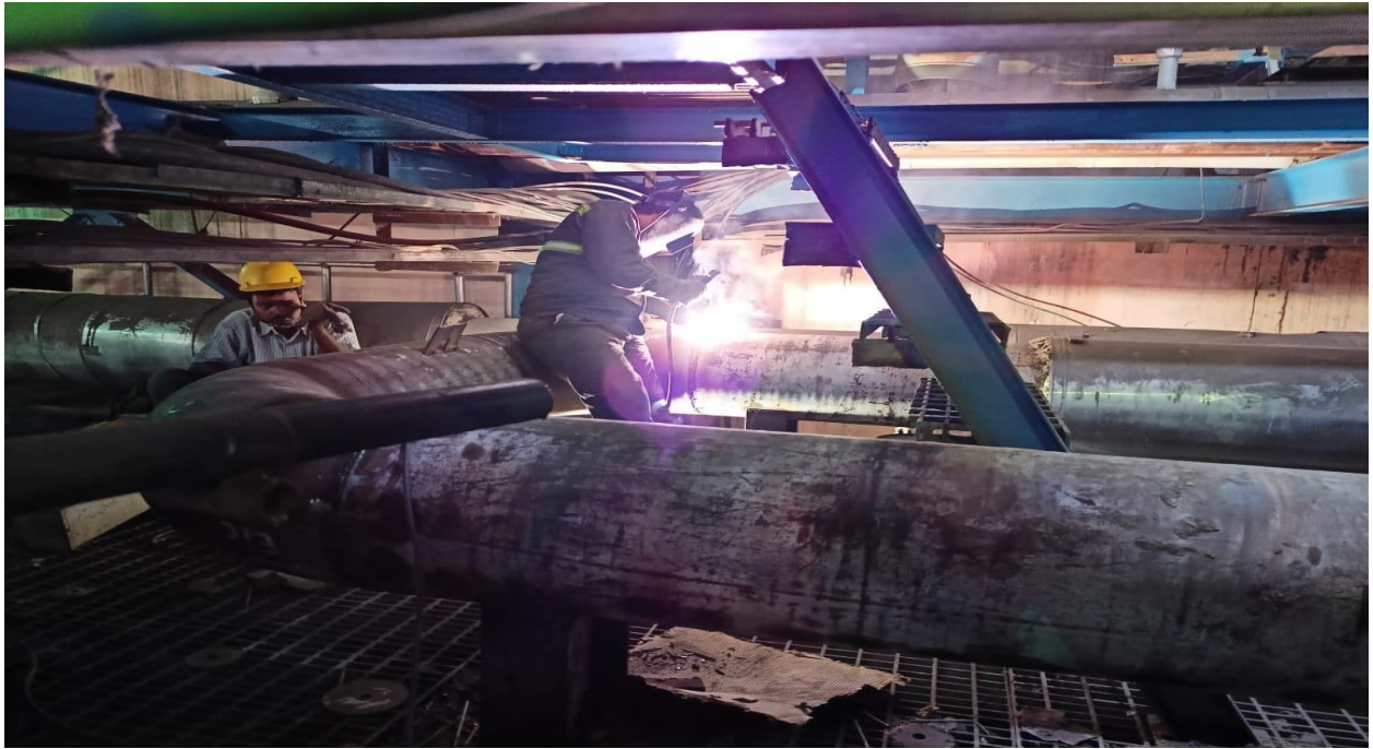
Figure 13: Final welding for joint-4 under progress
