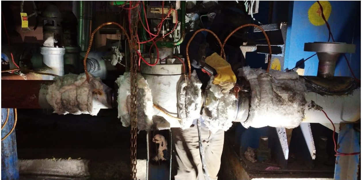
Figure 13: Preheating and root welding
