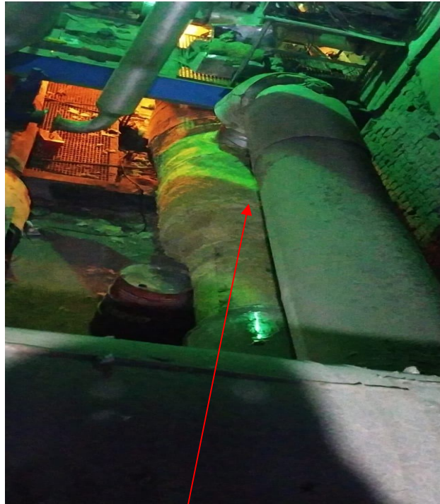
Figure 7: Insulation work after completion of PAUT
