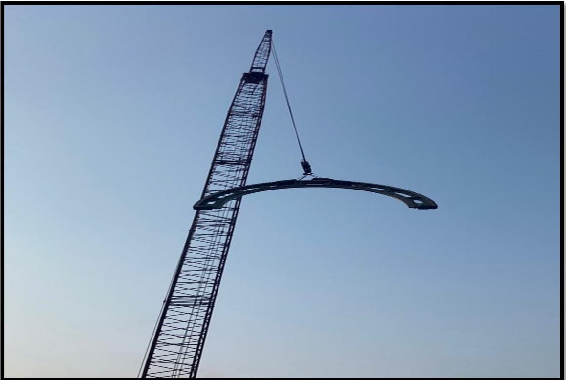
Existing girth gear dismantled.
