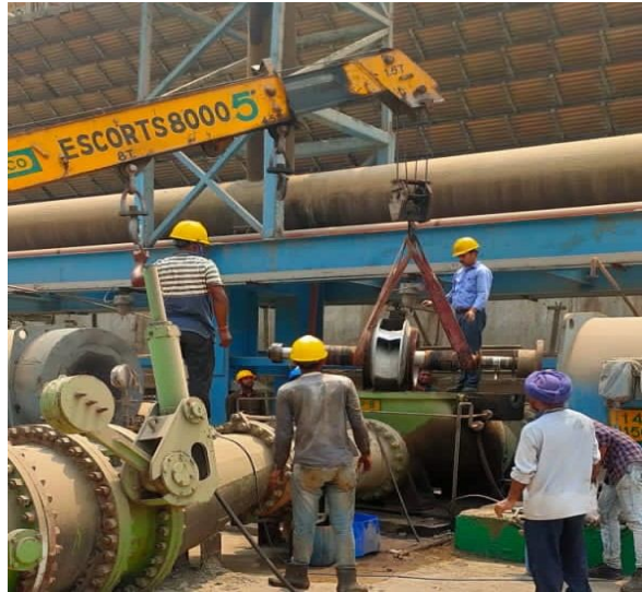
Rotor assembly during erection
