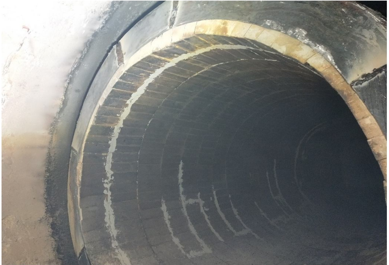
After refractory brick application
