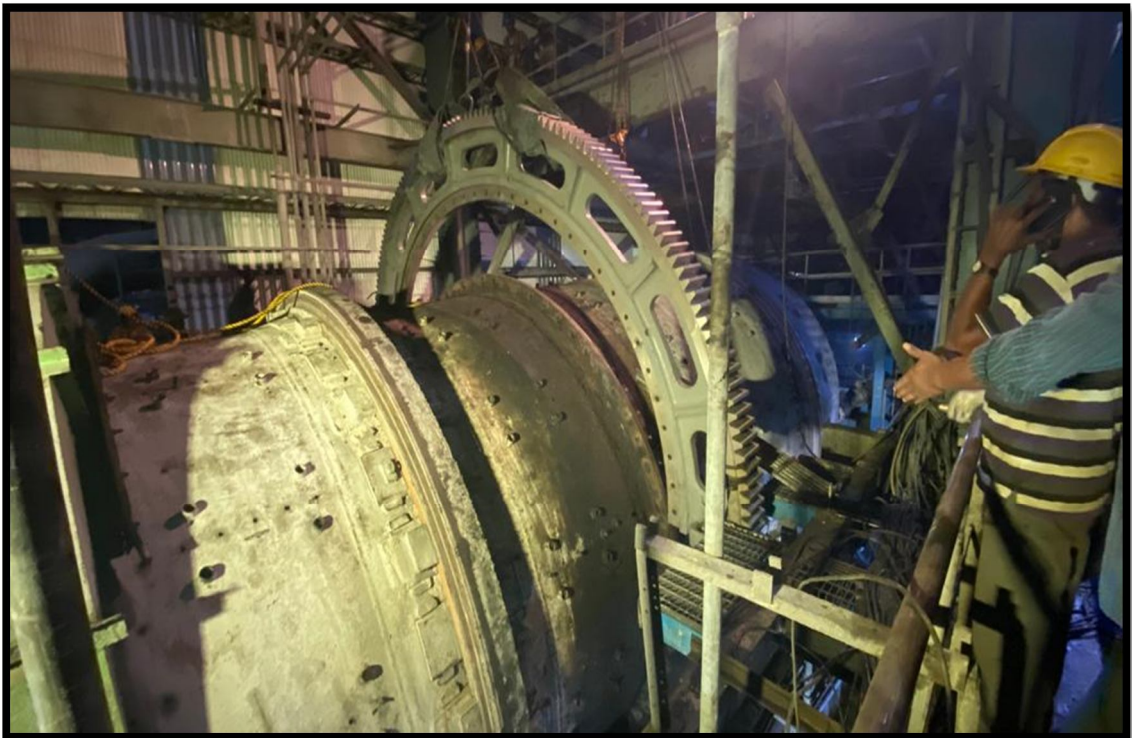
New girth gear erection
