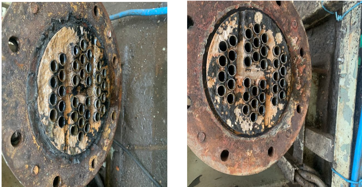
Fig 1.4.1(d) Lube oil cooler bfw turbine after cleaning
