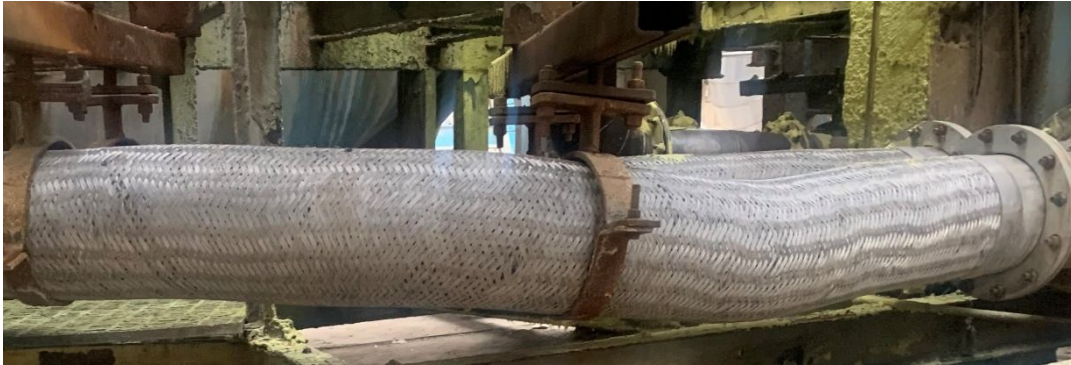
Fig 1(d) PA line Hose after replacement with new one
