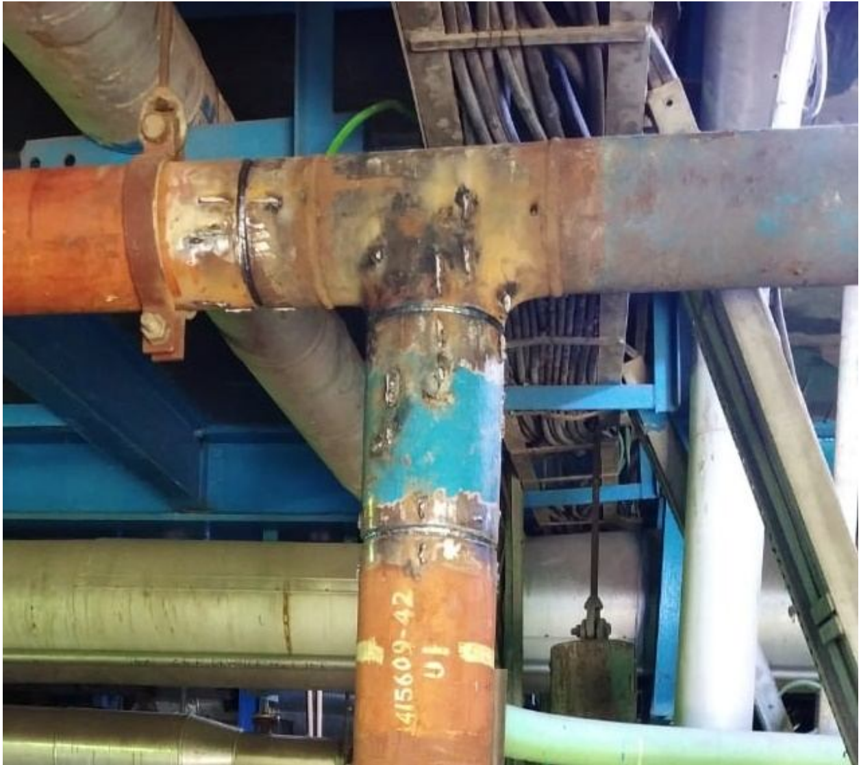
Figure 5: Root welding (TIG) completed
