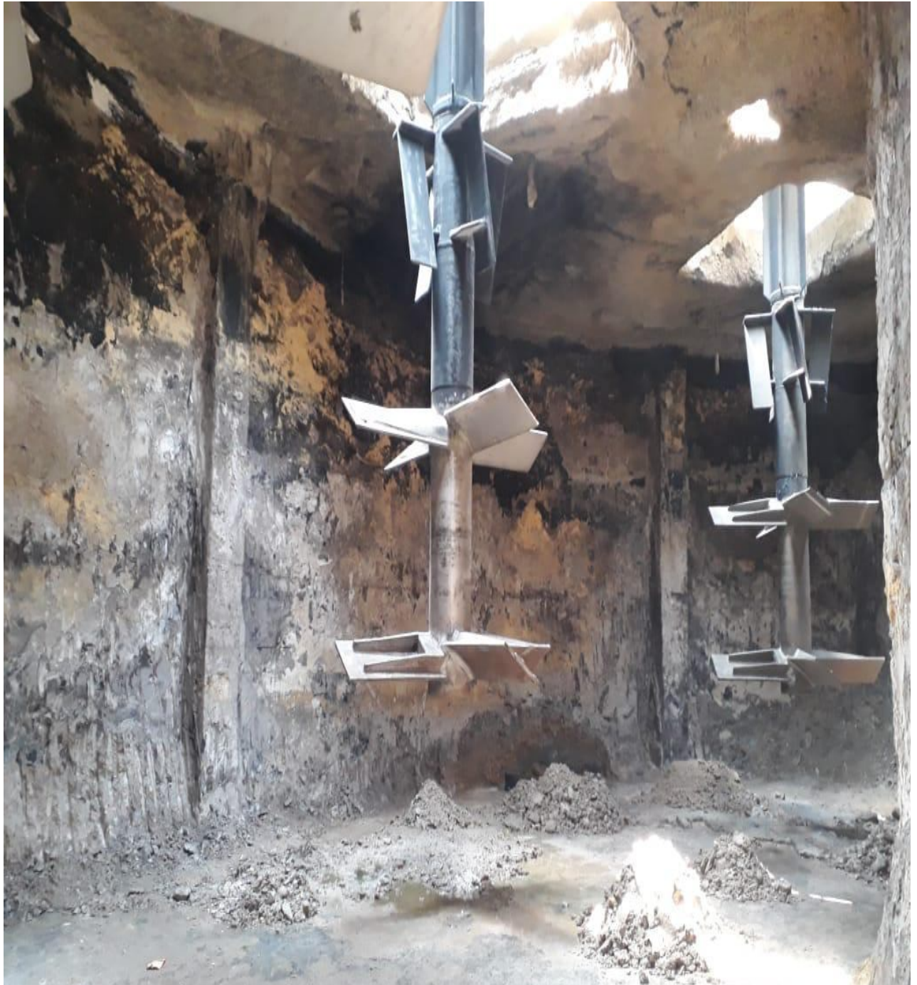
REPAIRED SPARE AGITATORS INSTALLED IN 05-113 & 05-114 LOCATION IN ANNULAR COMPARTMENT
