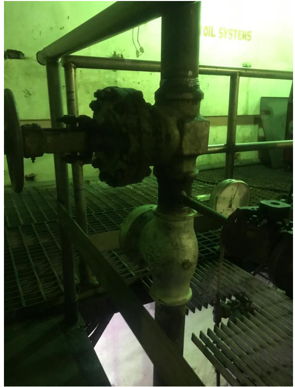
Figure 8: GOP(M) NRV after relocation & replacement
