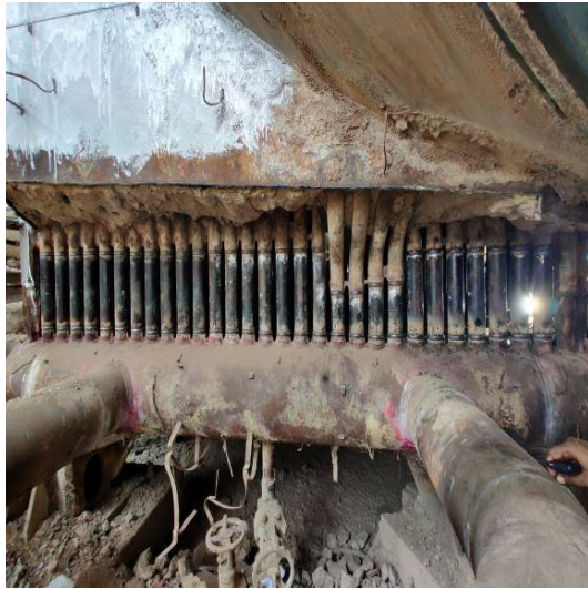
Boiler bypass nozzle top portion badly damaged which is replaced with new one.
