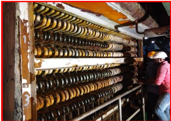
Thickness measurement carried out at various pr.parts in boiler
