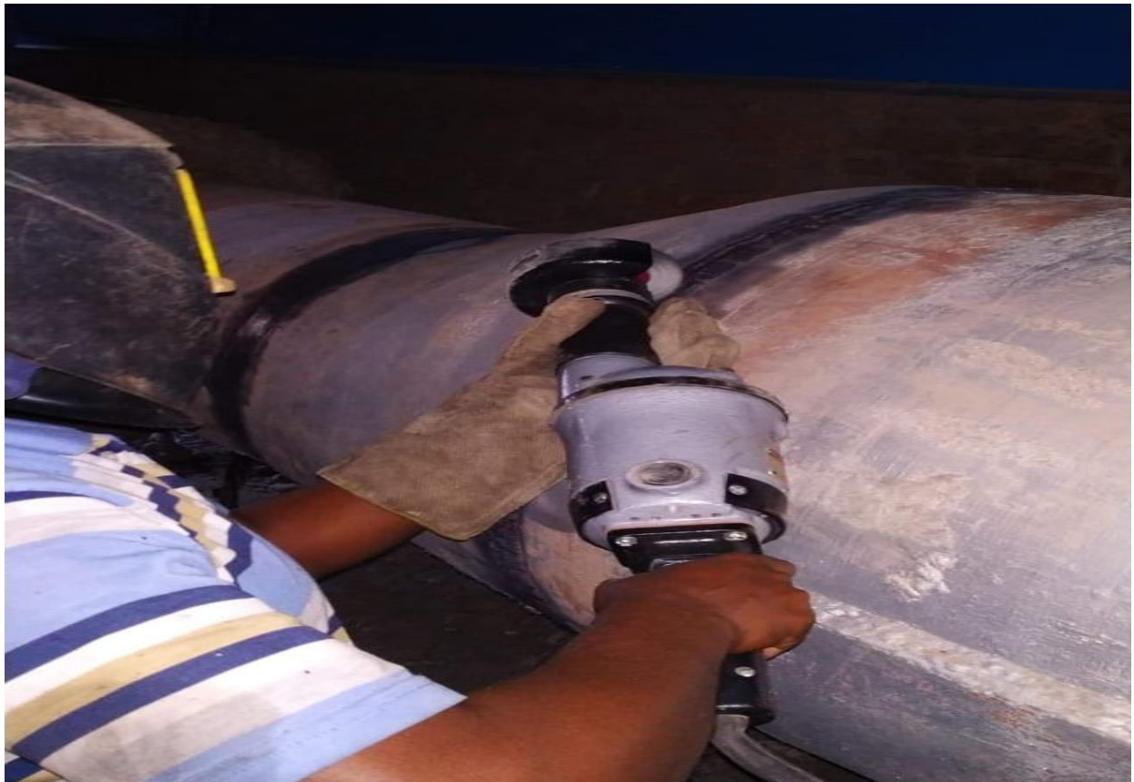
Figure 3: Joint surface cleaning under progress using buffing machine
