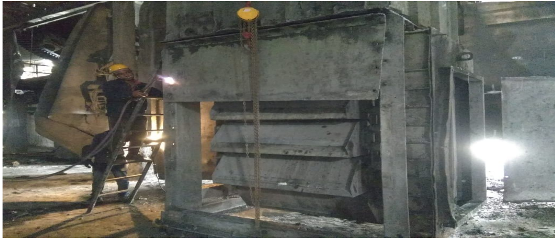
Primary elevator chain bucket inspection
