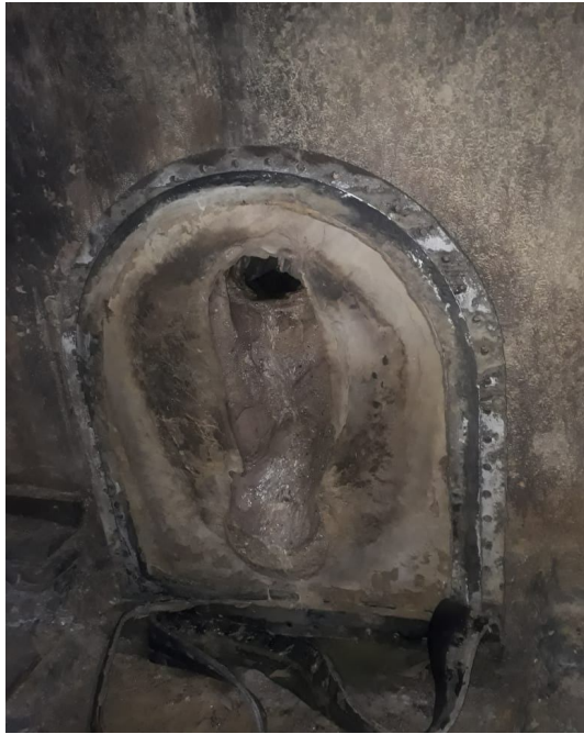
VCST manway before descaling
