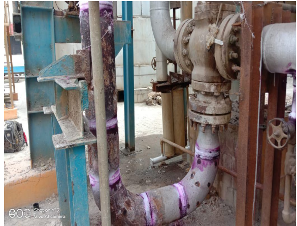
3 way valve joints DP test
