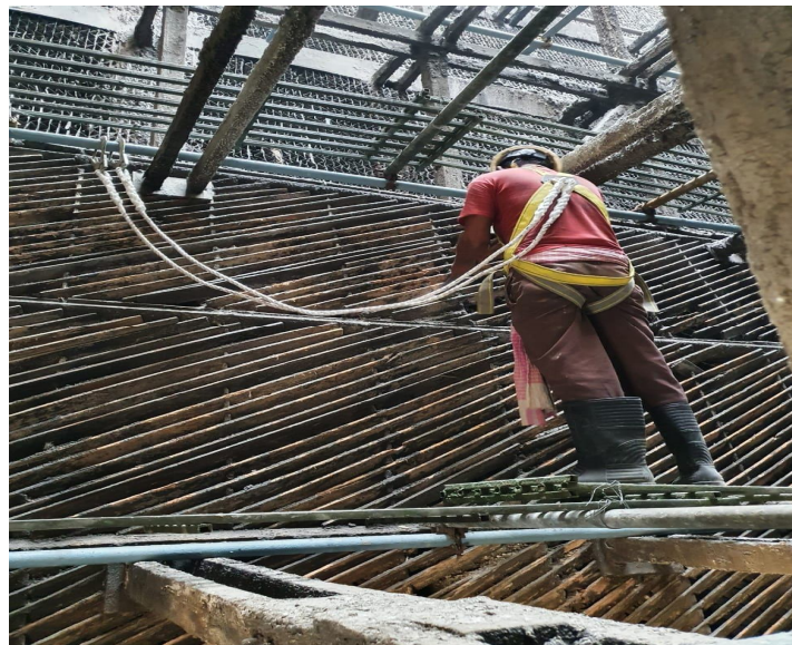
Old Cooling Tower mist eliminator cleaning
