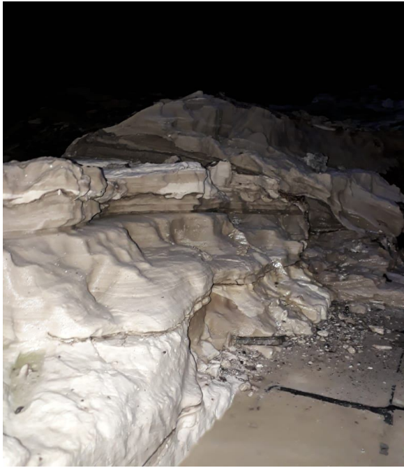
New pump tank before cleaning
