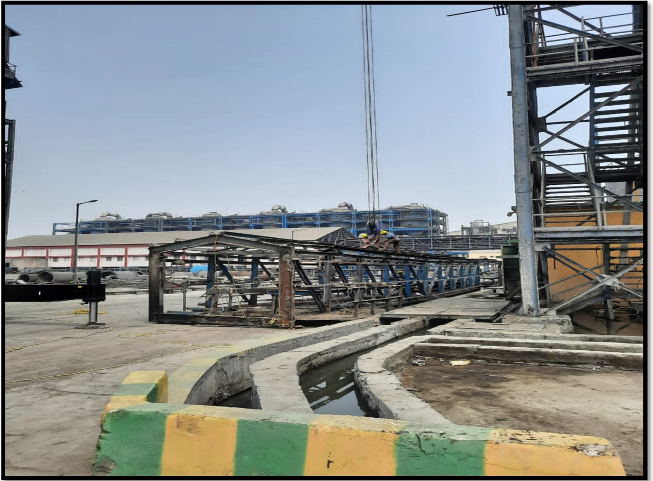
Product Conveyor gallery erection
