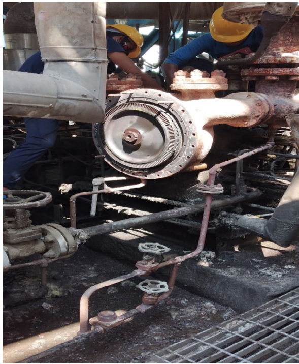
CWP TURBINE ROTOR DISMANTLE
