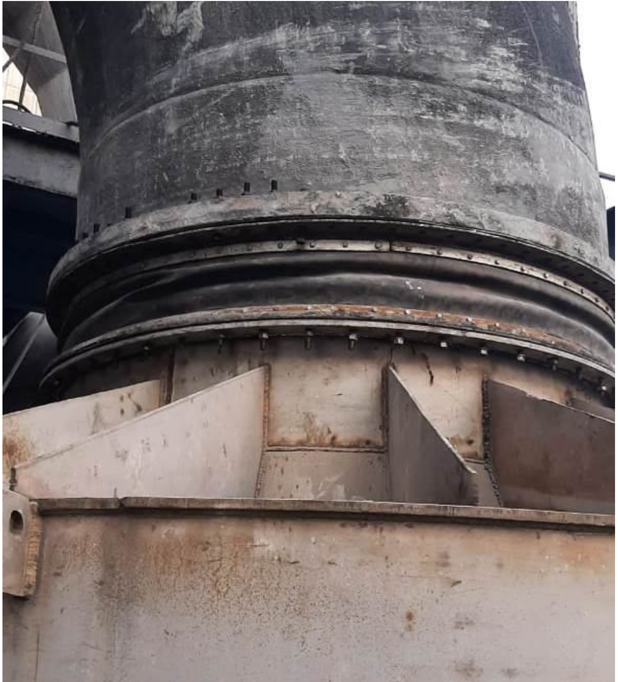
Prescrubber separator bellow replaced
