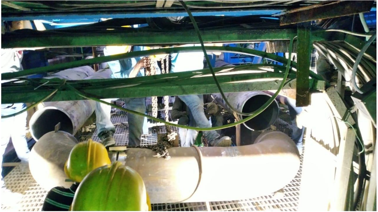
Figure 6: Elbow fit up under progress
