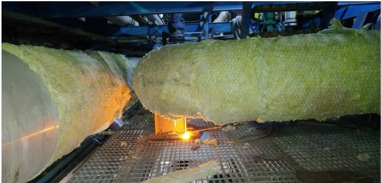
Figure 14: Header locking removal & insulation application
