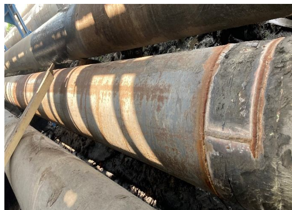
TG Cooling tower line Replacement after
