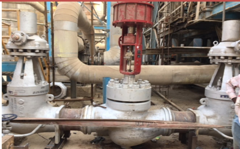
New Export steam Control Valve Tag 10PCV1304
