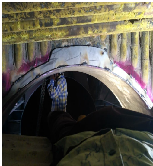
Boiler bypass nozzle top portion badly damaged which is replaced with new one.
