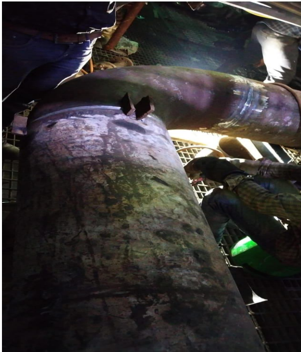
Figure 7 & 8: Both Elbows are fitted and ready for welding
