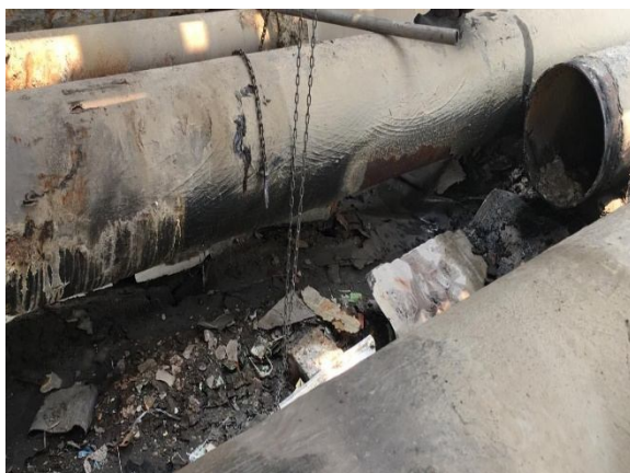
TG Cooling tower line Replacement before
