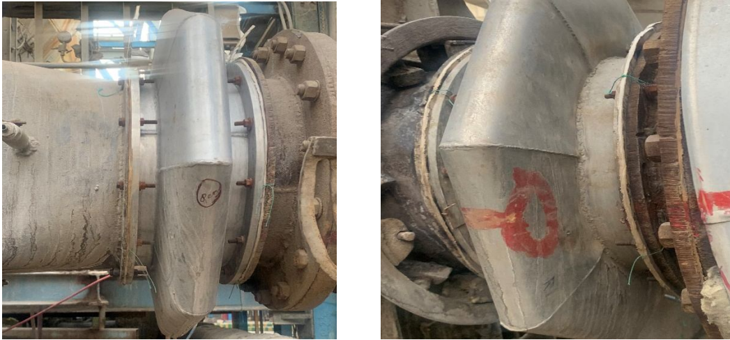
Fig 2.2(b) Suction and discharge bellow after replacement with new one
