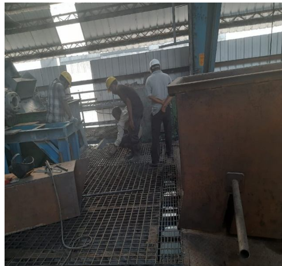
Discharge diverter fabrication
