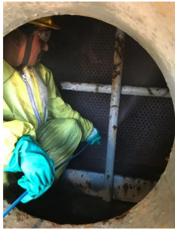
Hydro jet cleaning
