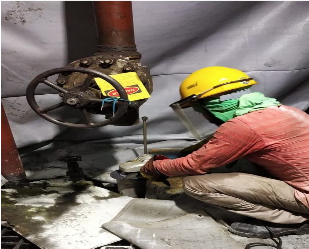
Figure 4: GOP(S) discharge pipe edge preparation is under progress
