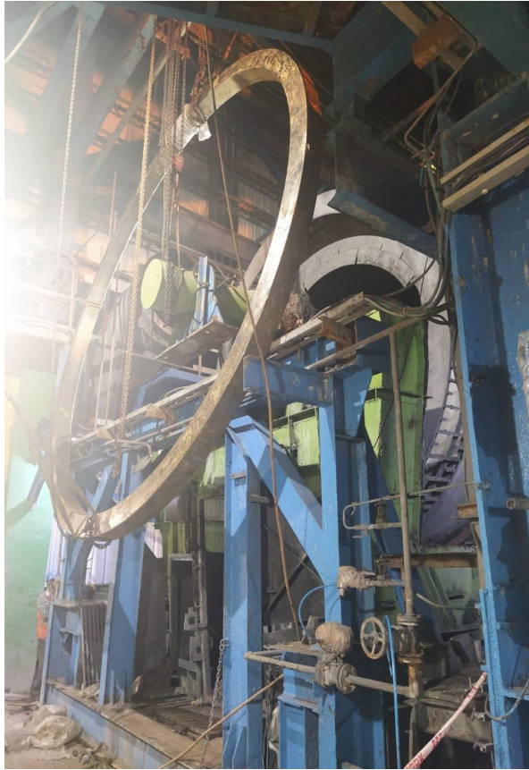
Discharge end tyre fitting
