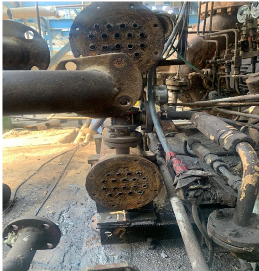
Fig 1.4.1(e) lube oil cooler of bcw turbine before and after cleaning
