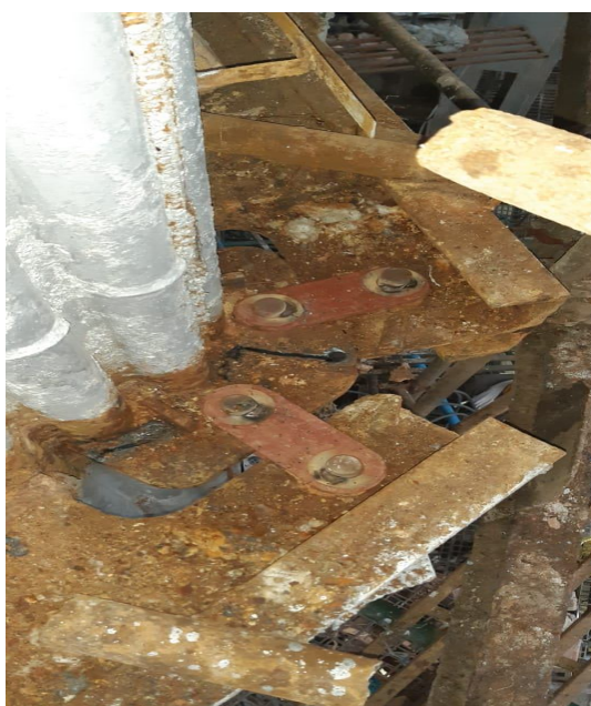
Various pictures of Buck stay corner plate modified at various elevations
