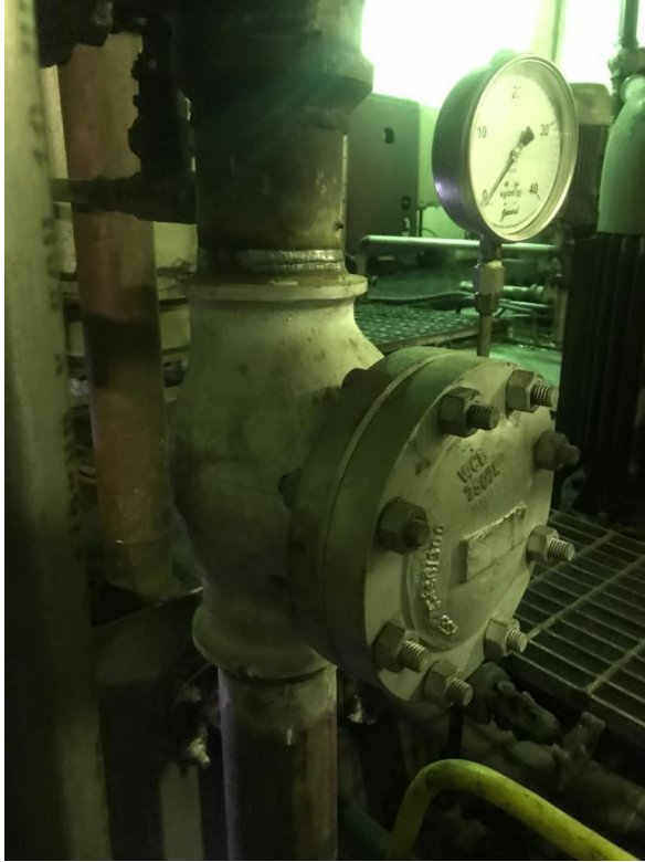
Figure 7: GOP(S) NRV after replacement
