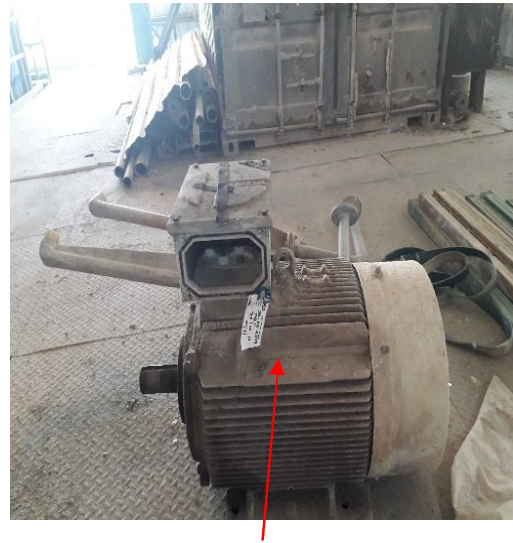
Old Removed out Motor
