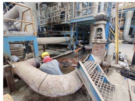
Removal of valves
