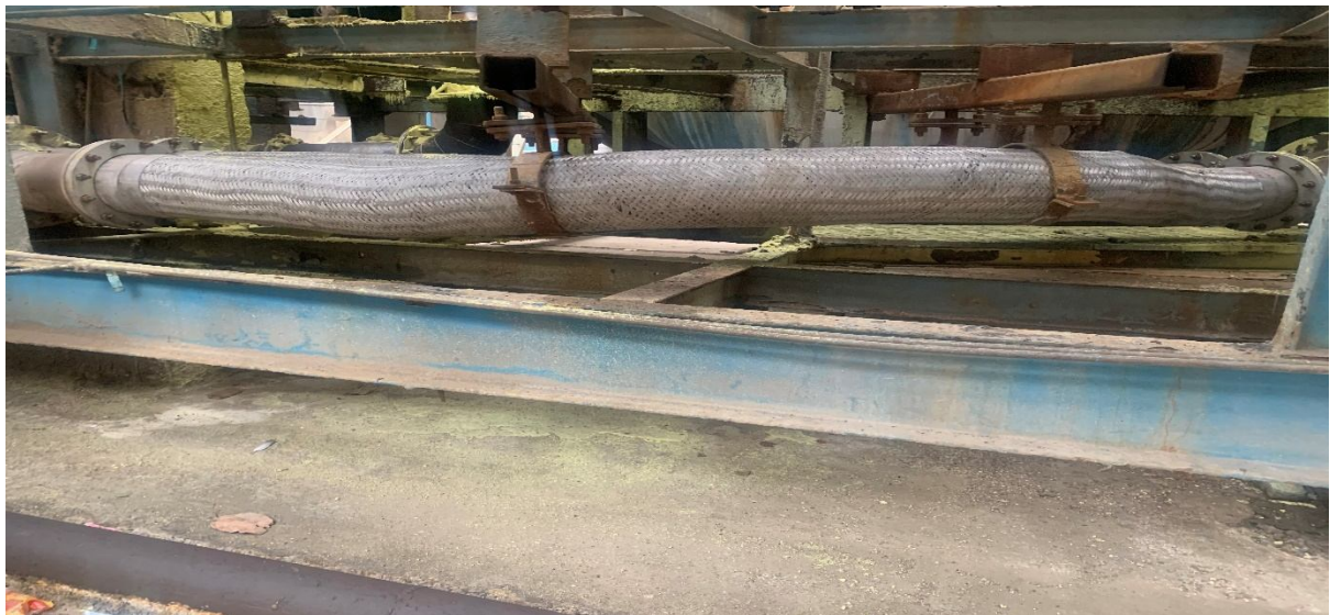
Fig 1.1(e) PA line Hose after replacement with new one
