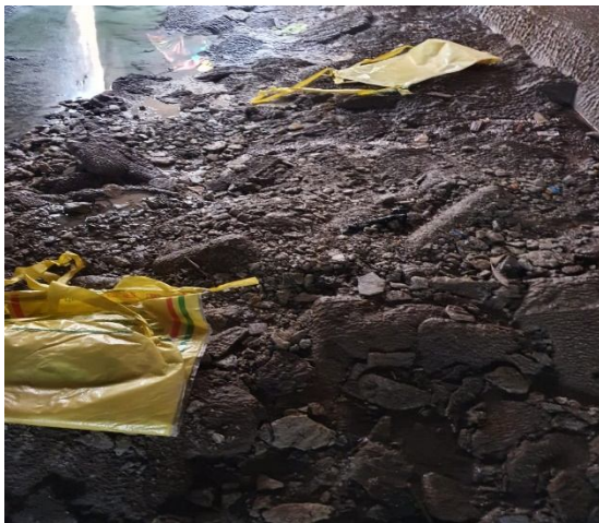
Hot well trench before cleaning
