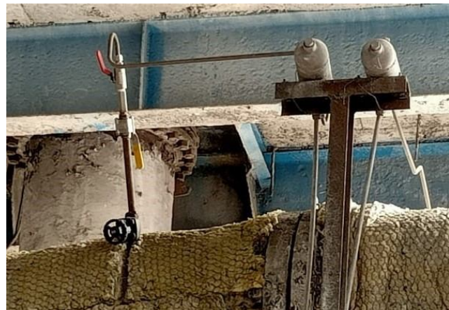
New Root isolation valves of Orifice tapings
