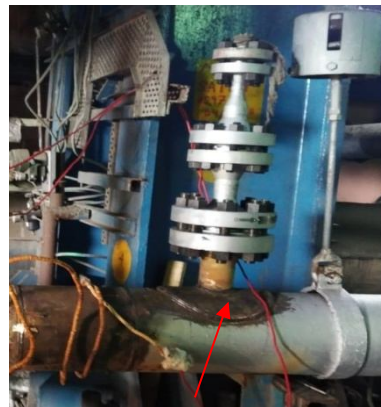
Figure 7: Branch joint pad is welded
