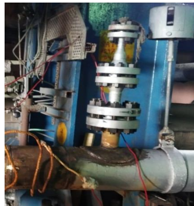
Figure 7: Branch joint pad is welded
