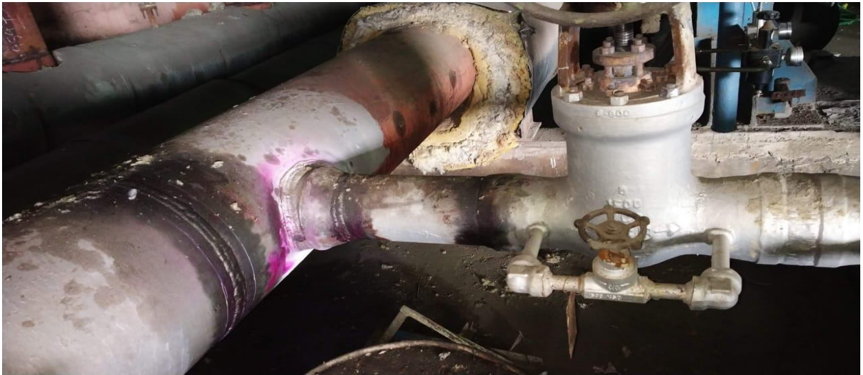
Figure 5: PAUT completed joints
