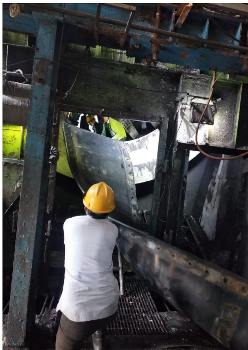
EPDM Panel replacement
