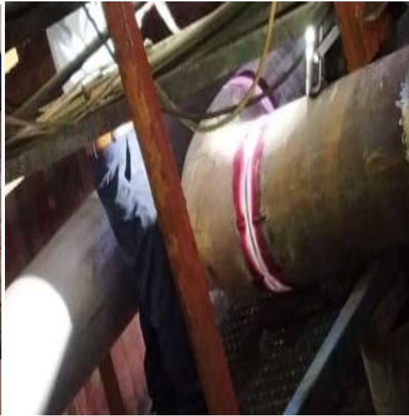
Figure 12: DP test for Joint-3 & 4 roots welding
