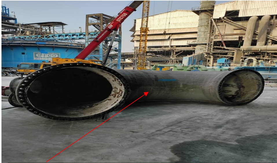
U- DUCT DISMANTLED FOR CLEANING PURPOSES.
