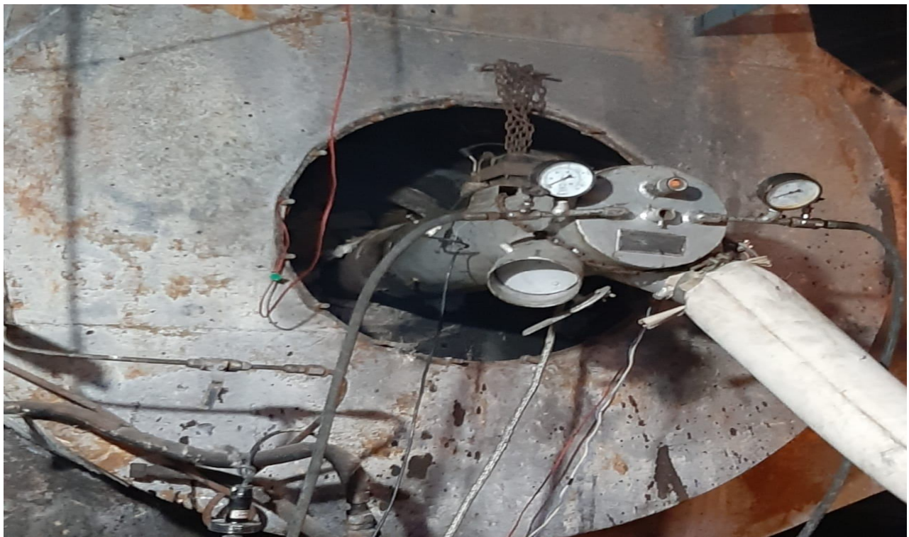
Heat dryout process after refractory application
