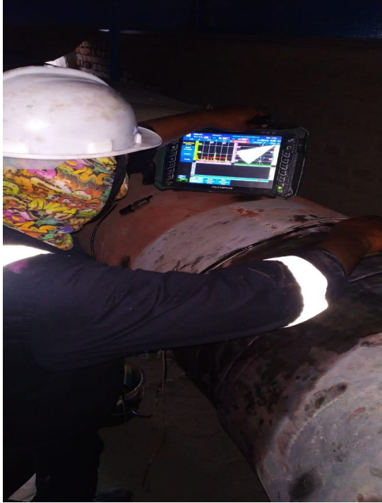
Figure 6: PAUT of joint under progress
