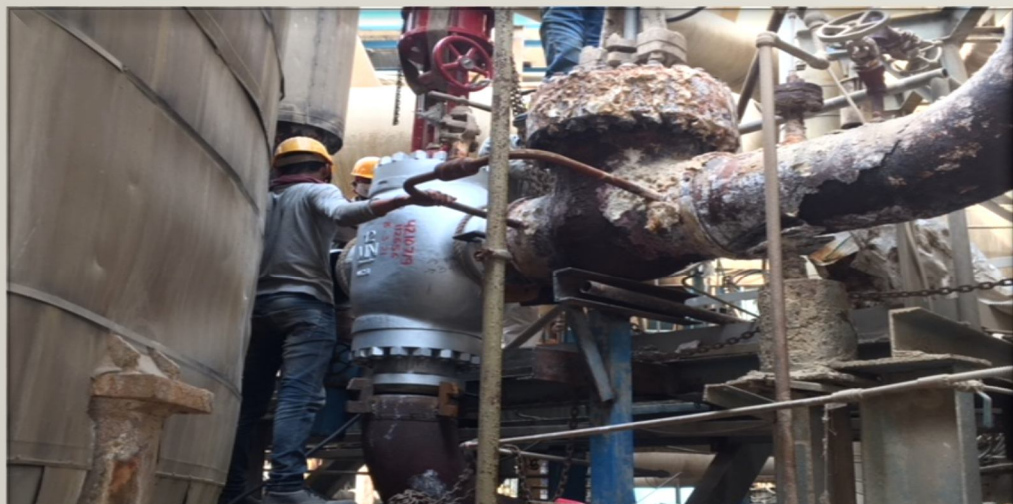
New 3-Way 10TCV1506 after Replacement
