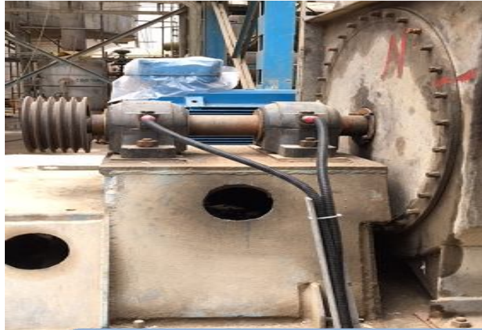
Vibration Probe installation In PA Fan
