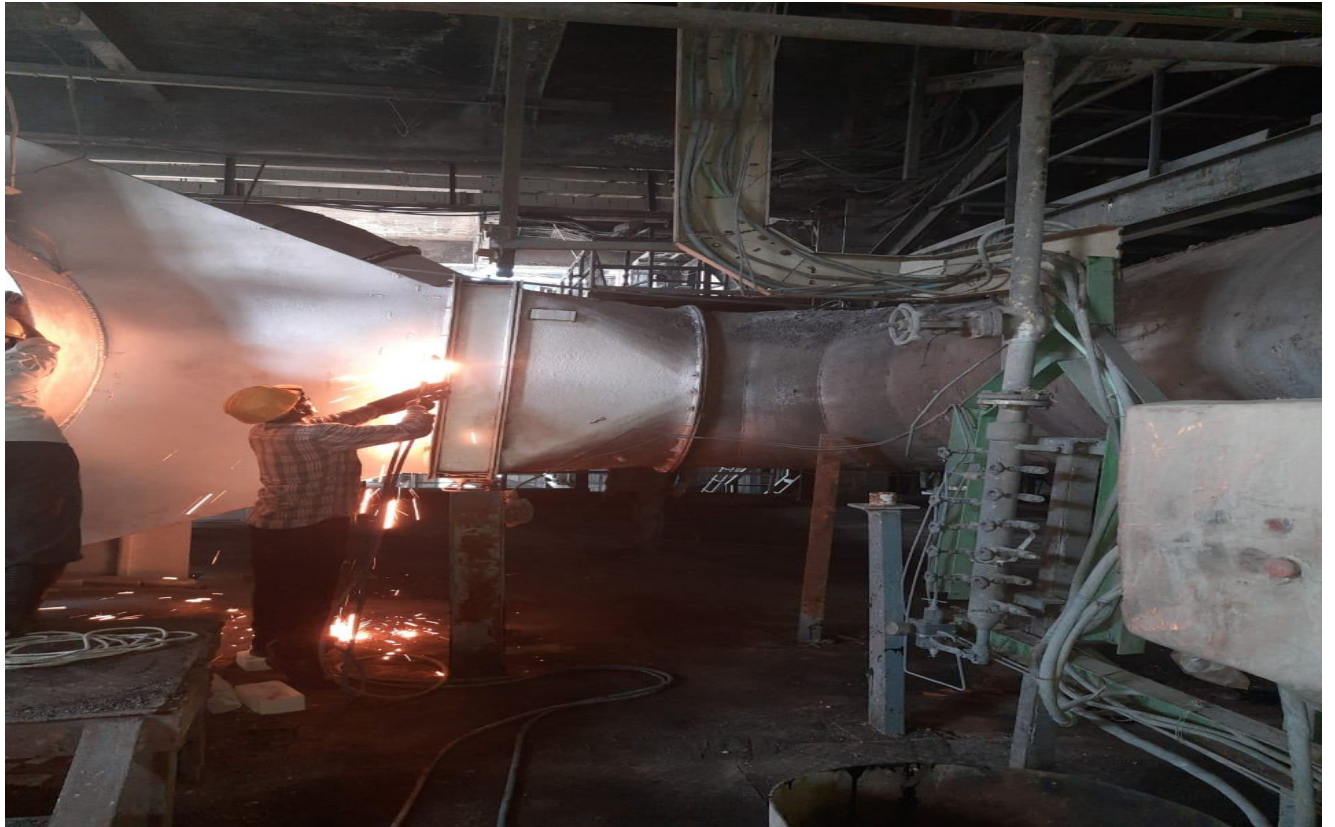
Quench air fan discharge damper replacement under progress.
