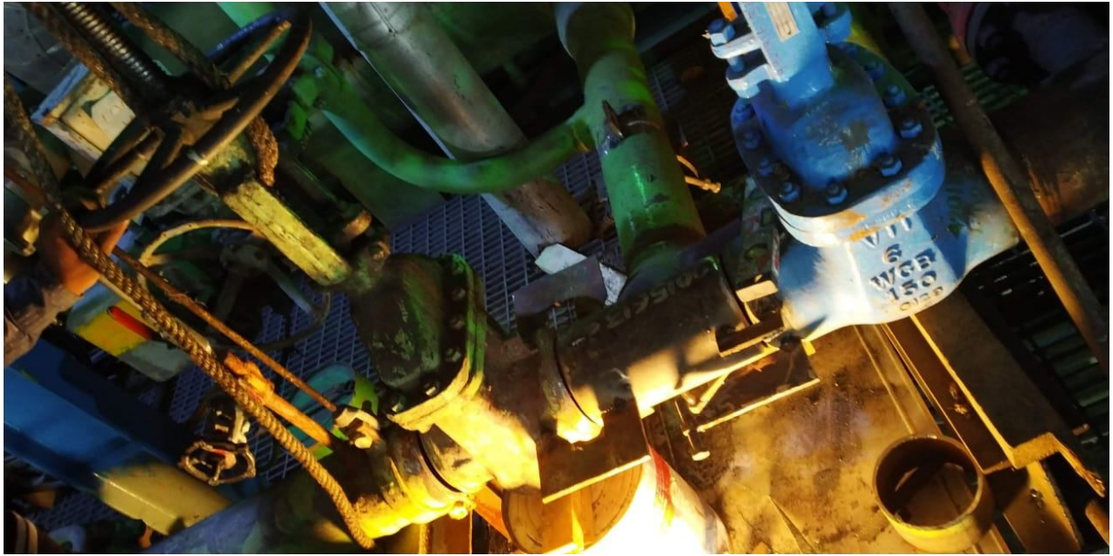
Figure 3: 150 NB joints fit up job is under progress
