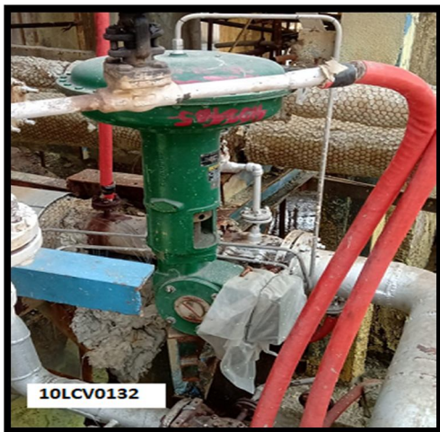
Control valve after Re-location
