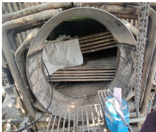
Boiler bypass nozzle top portion badly damaged which is replaced with new one.
