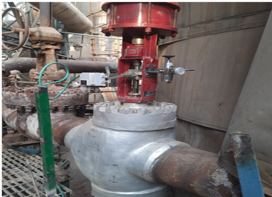
New 3-Way Control Valve 10TCV2506
