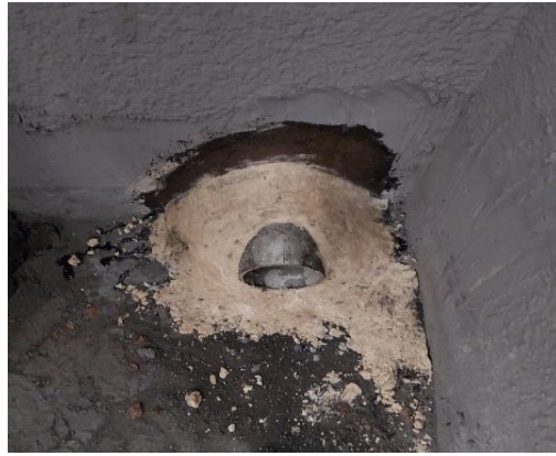
Grouting of S.S. pipe
