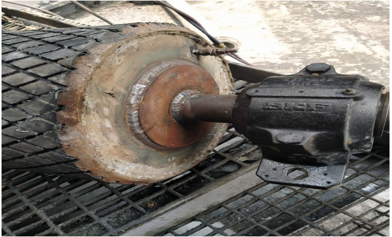
Tail pulley pad plate welding
