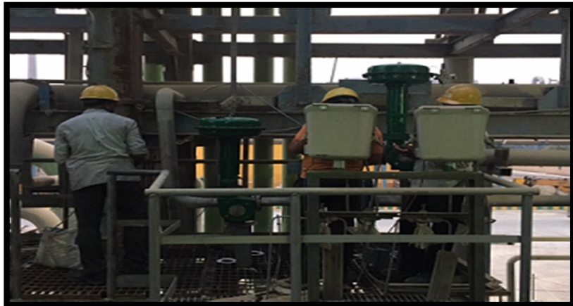
Control Valve replaced for 10AV2450, 10LV2440
