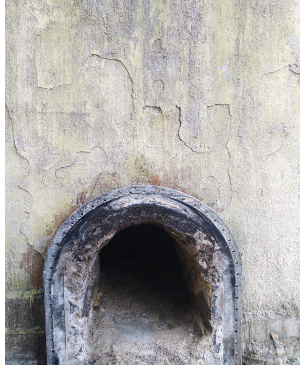
Annular Manway after cleaning
