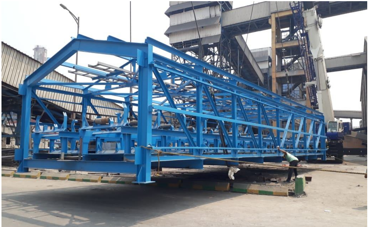
NEW GALLERY FOR ERECTION
