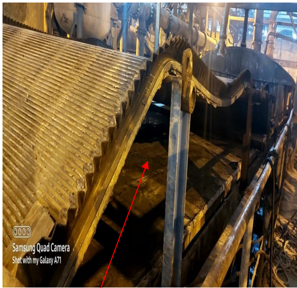
Top Cover replacement job
