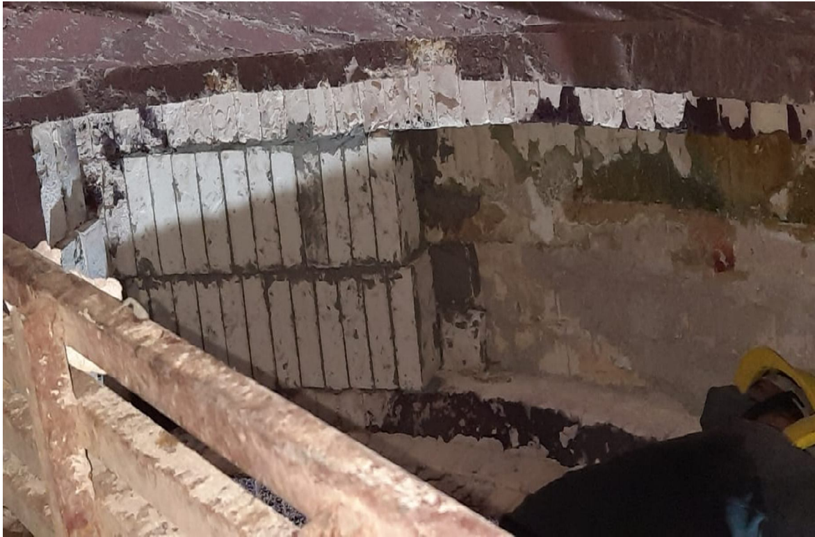
Brick lining work of furnace to dished head area
