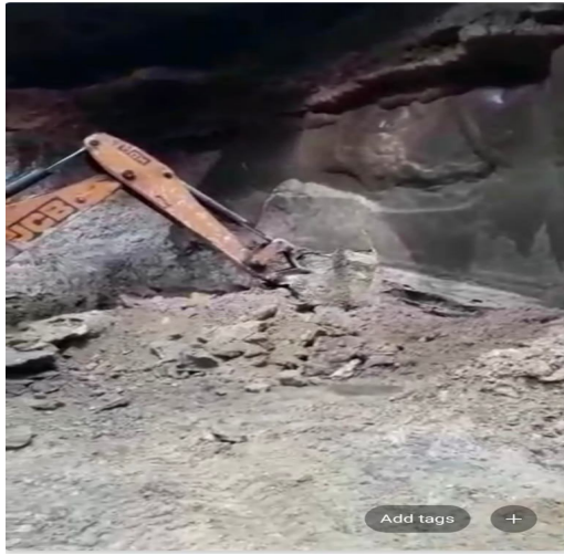
Reactor annular section inside cleaning with JCB
