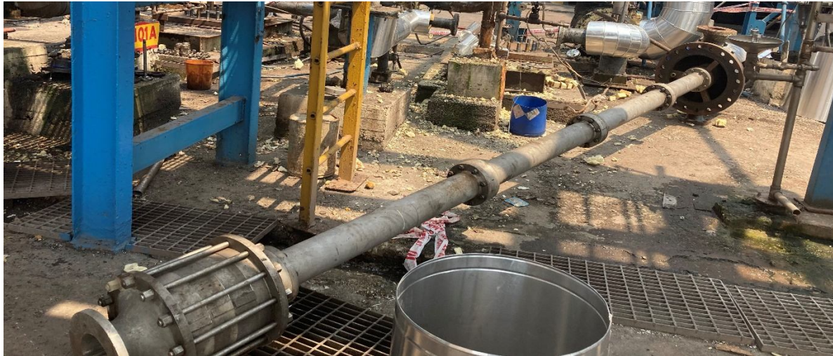
Ammonia transfer pump B ready for erection.
