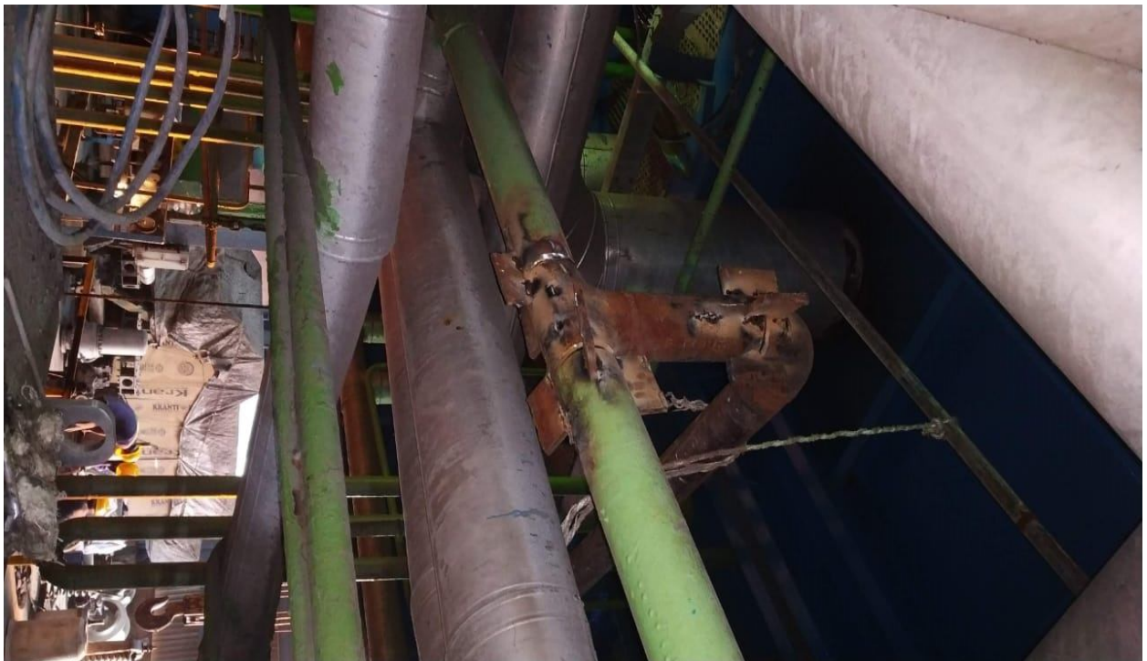
Figure 4: 80 NB pipe fit up completed
