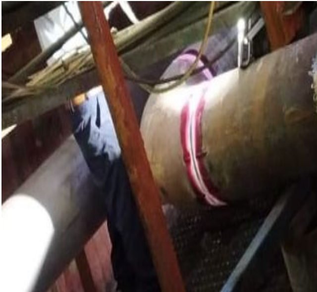
Figure 12: DP test for Joint-3 & 4 roots welding
