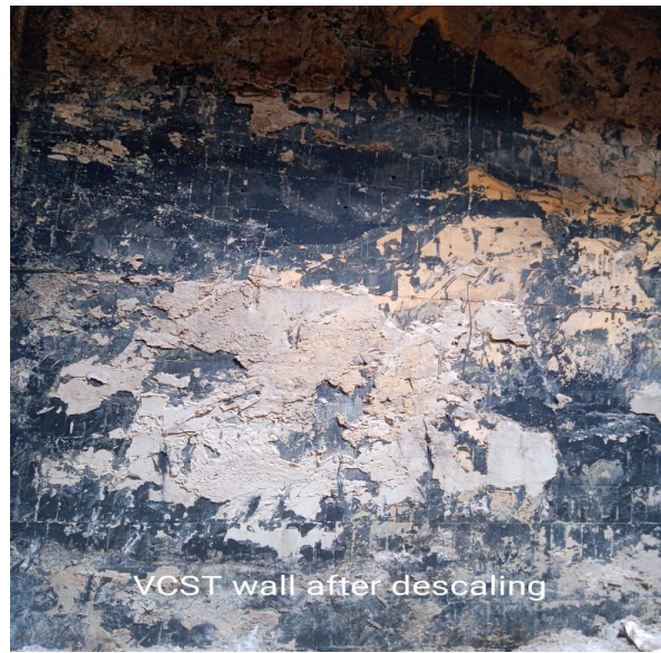
VCST wall after cleaning
