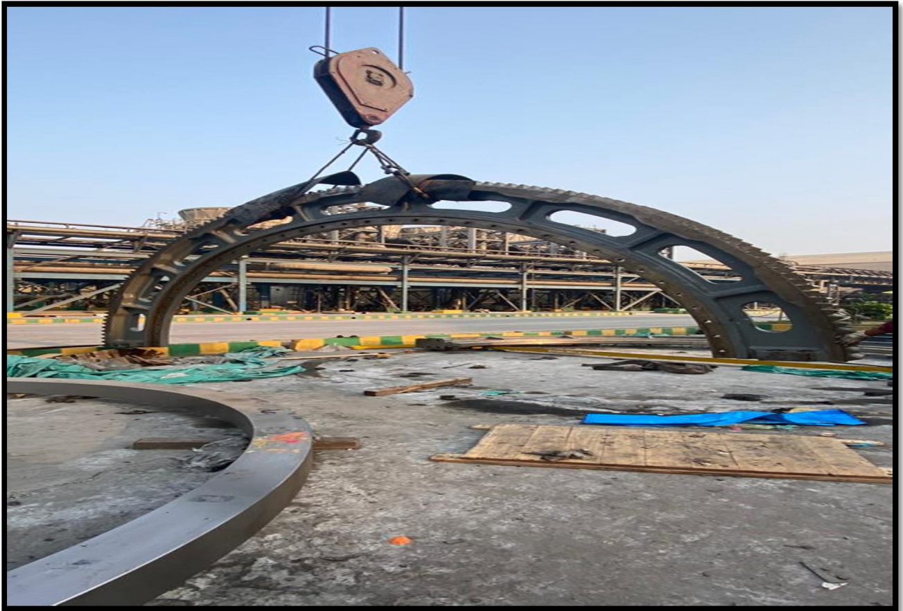
New girth gear shifting.
