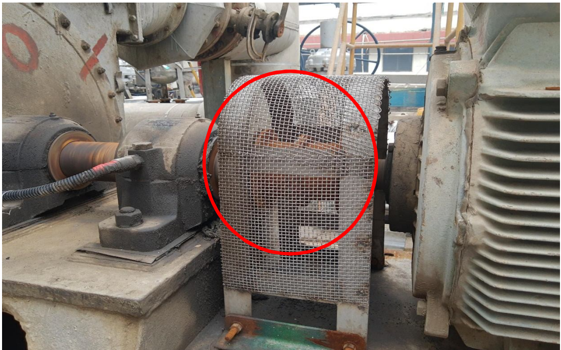
Fig 2.2(c) PA fan from pulley drive to direct coupling
