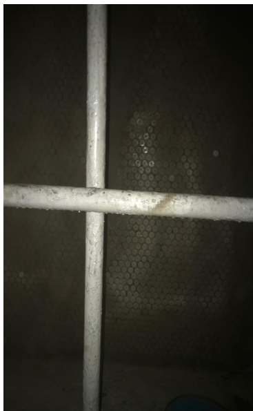
After sand blasting
