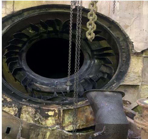
Fig 2.1(a) damaged vane of air resister fig 2.1(b) after vane replacement
