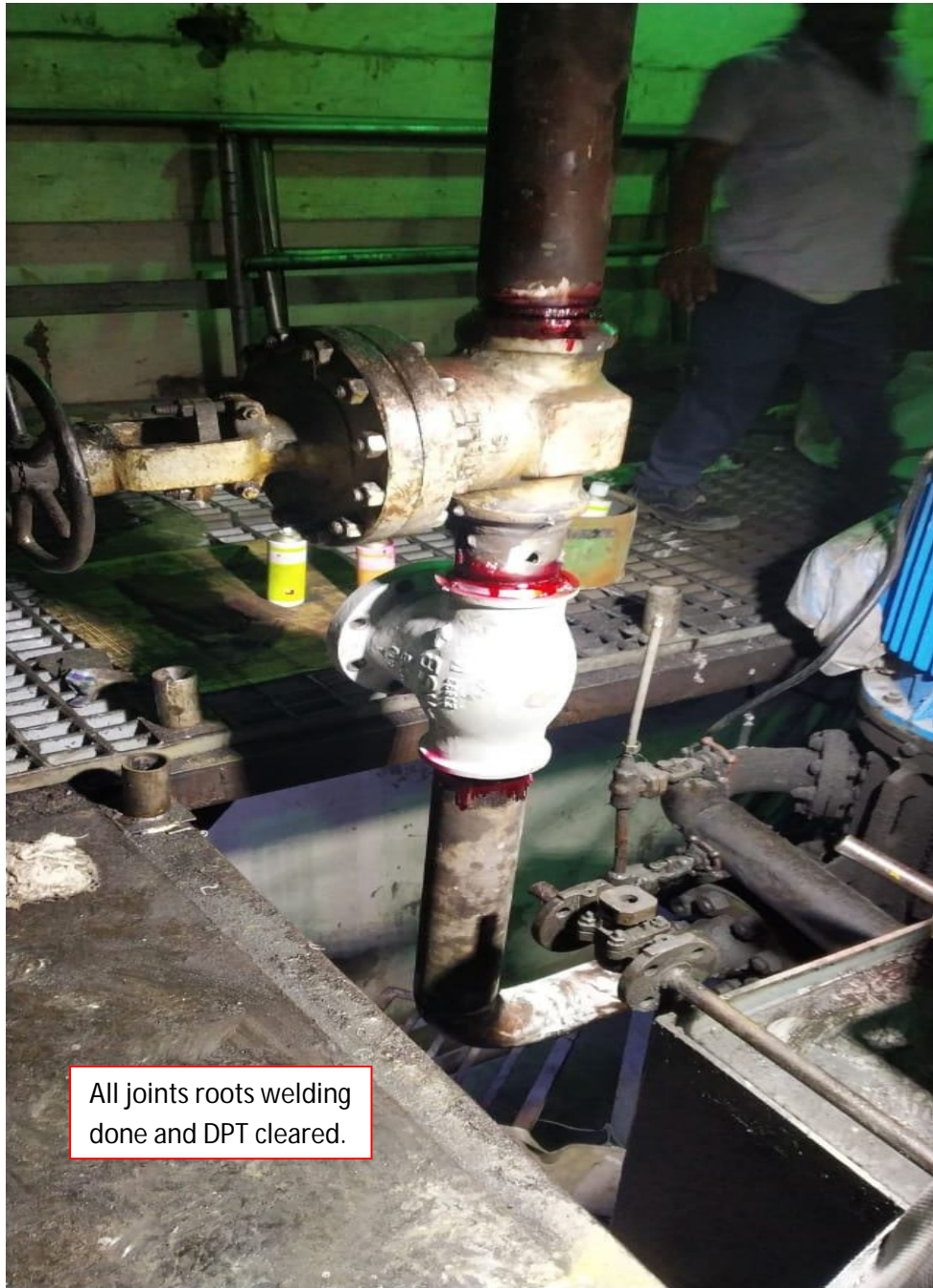
Figure 6: GOP(M) NRV replaced and Valve & NRV relocated
