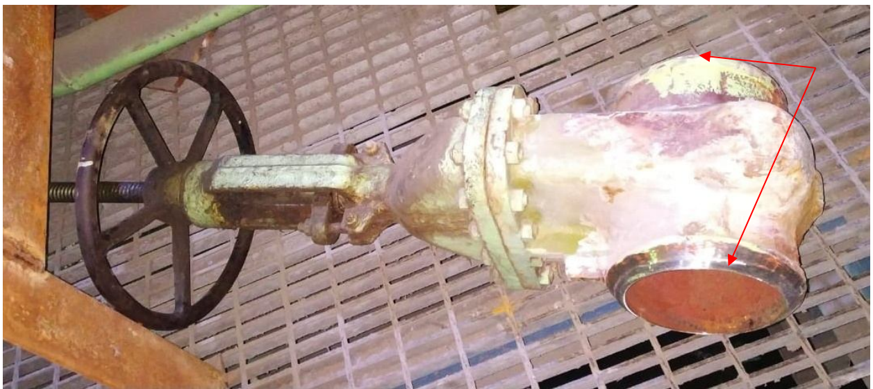
Figure2: Old valve edges are prepared
