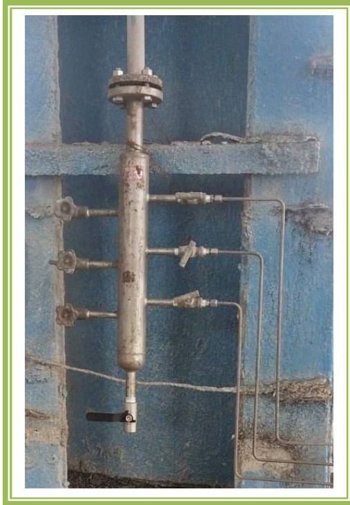
New Instrument Air Manifolds in Evaporator area
