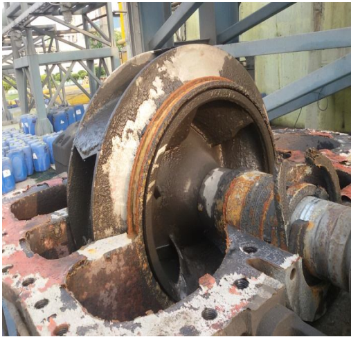
Rotor Assembly Condition after top casing removal
