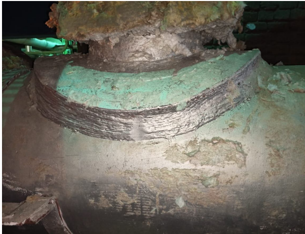
Figure 2: Insulation removed from HP steam header
