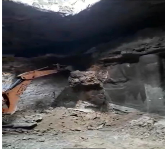
Reactor annular section inside cleaning with JCB
