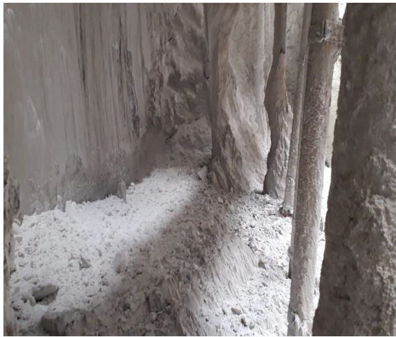
Fumes scrubber chamber before cleaning
