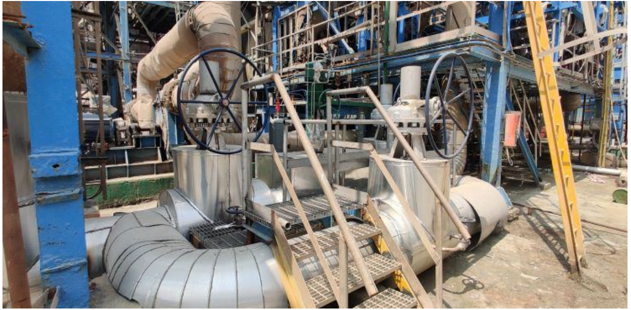
AFTER INSULATION AND PLATFORM INSTALLATION
