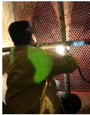
Inspection of cleaning
