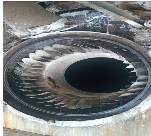
Fig 2.1(a) damaged vane of air resister fig 2.1(b) after vane replacement
