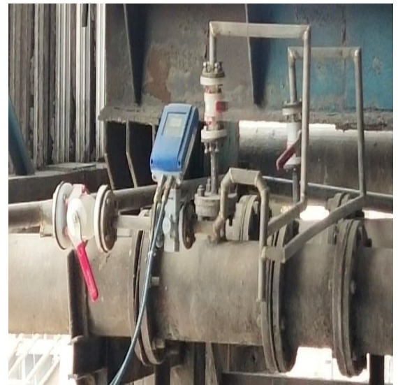
M/s Krohne Marshall make Electromagnetic Flowmeters in Flocculent lines
