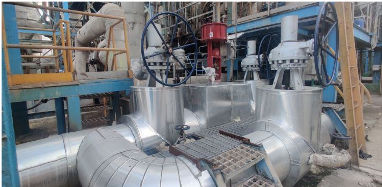
AFTER INSULATION AND PLATFORM INSTALLATION
