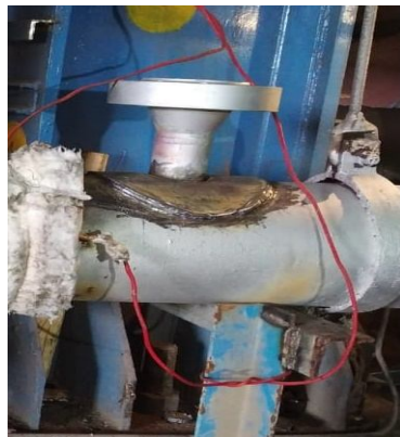
Figure 6: Branch joint pad fitted
