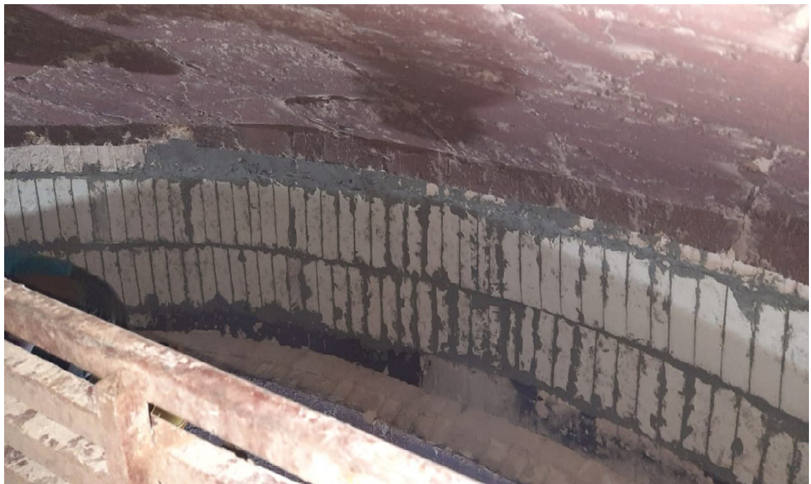
Brick lining work of furnace to dished head area
