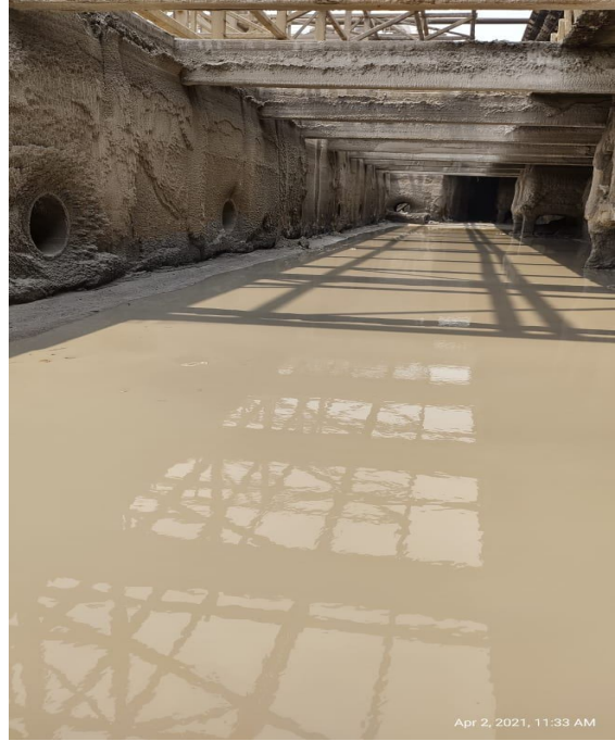
Old Cooling Tower Cell after cleaning
