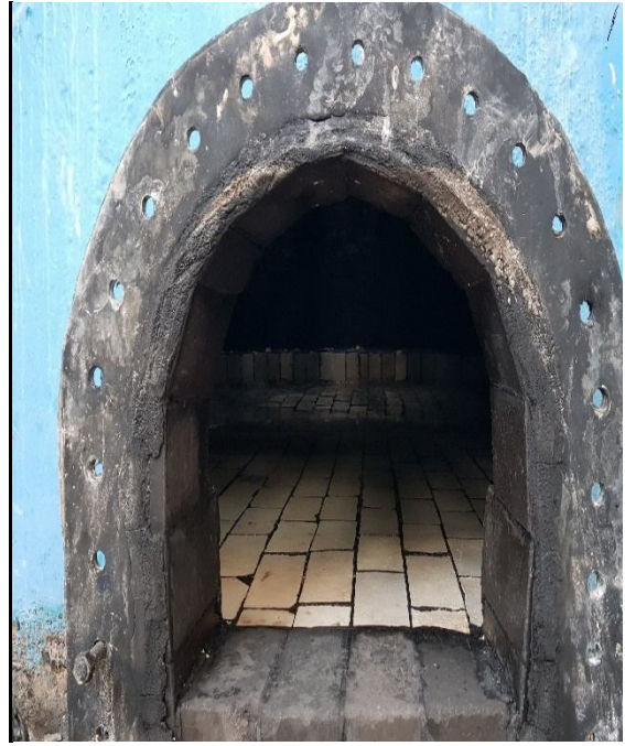
New pump tank after
