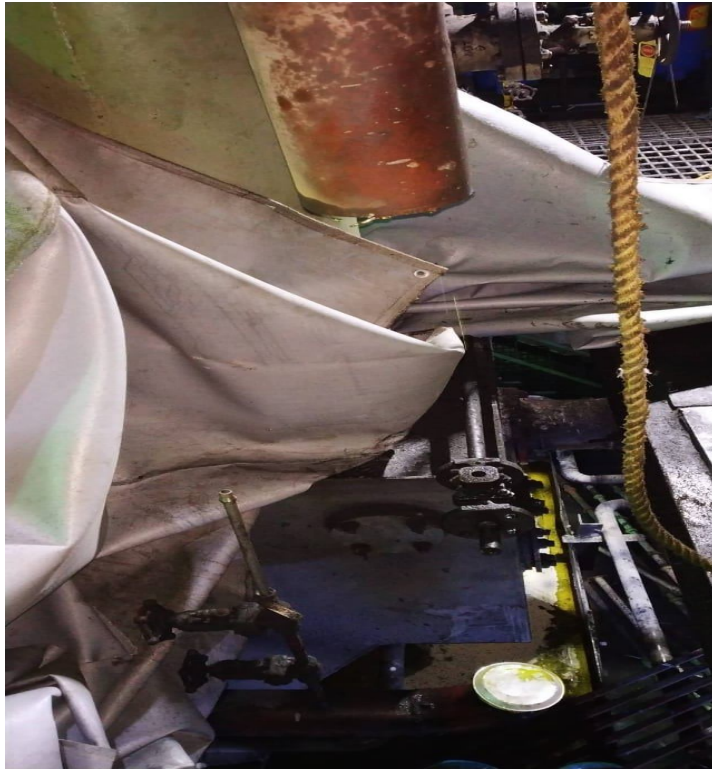
Figure 2: GOP(M) header after cutting NRV & valve
