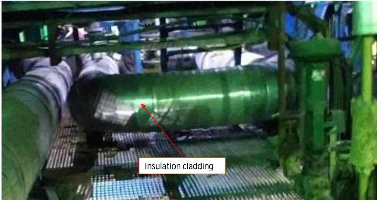
Figure 15: Insulation completed
