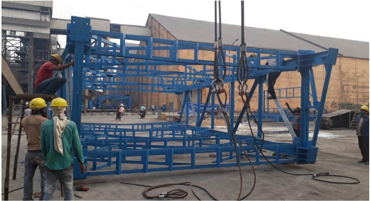
ALL NEW GALLERIES – 1 & 2 ALONG WITH TRESTLE NO-1 & 3 AFTER ERECTION:
