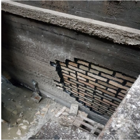
New Cooling Tower cold well cell wall repairing
