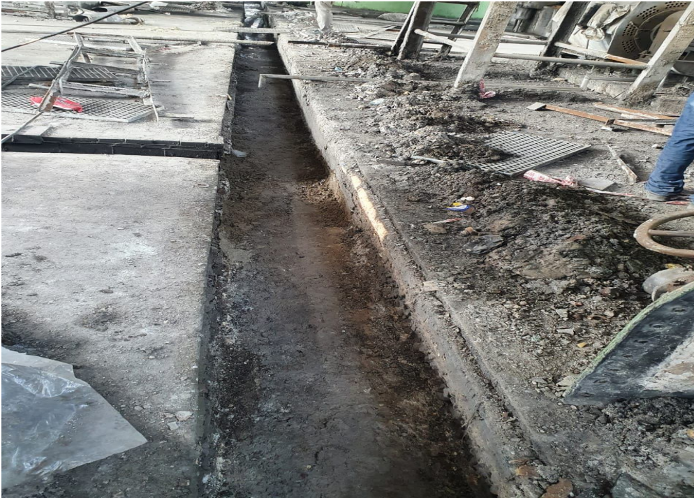
Evaporator area drain cleaning
