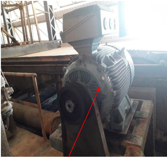
New Motor installation
