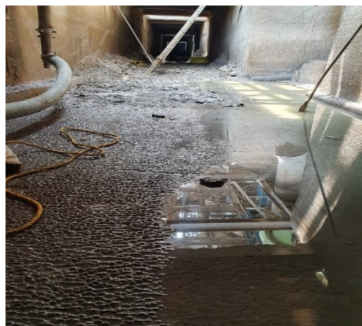
Hot well trench after cleaning
