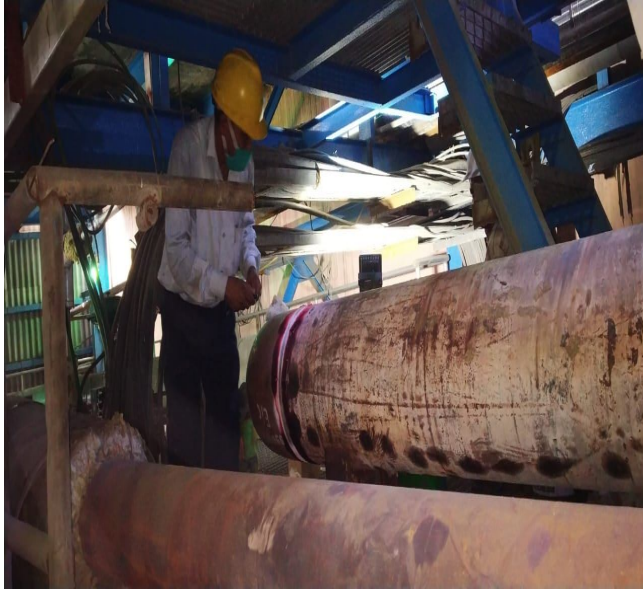
Figure 11: DP test for Joint-2 root welding
