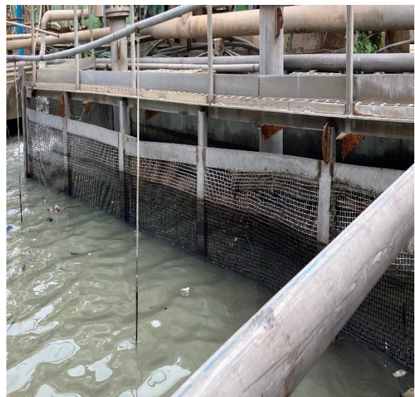
Neutralization pit pump suction strainer after replacement.
