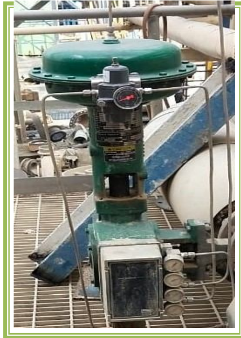
New M/s Fisher make Cloth was steam Control Valve
