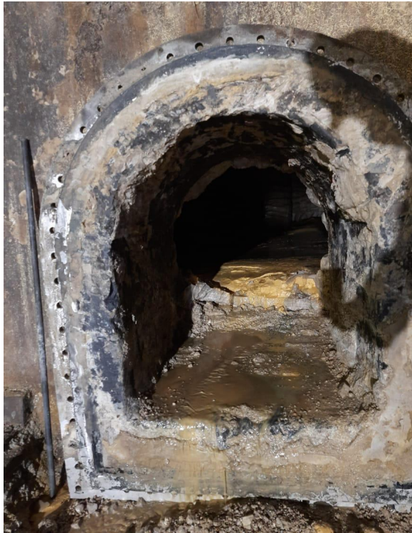
Annular Manway before cleaning
