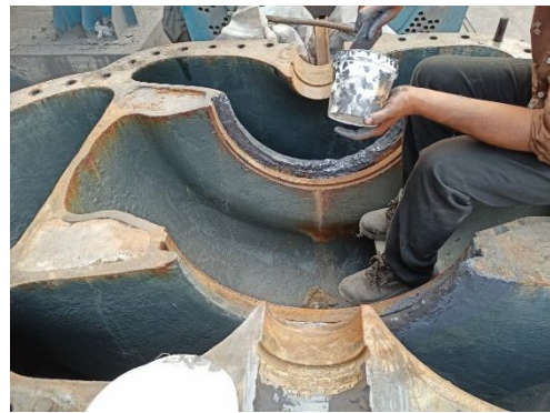
REPAIRING OF CASING
