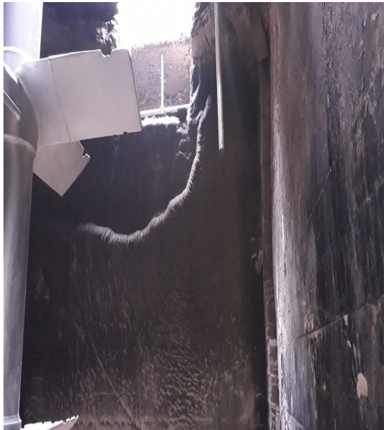
Adjustment tank wall before cleaning
